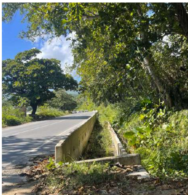
Figure 6-10: Concrete swale (u-drain) along coastal highway, East of Rozelle Falls
