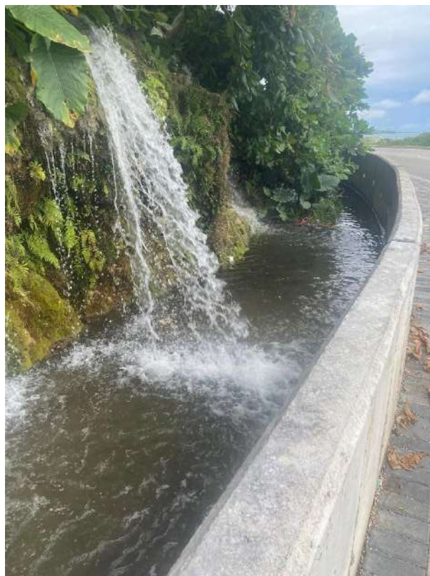
Figure 6-11: Concrete swale (u-drain) receiving stormwater discharges and overflow from the Rozelle Falls
