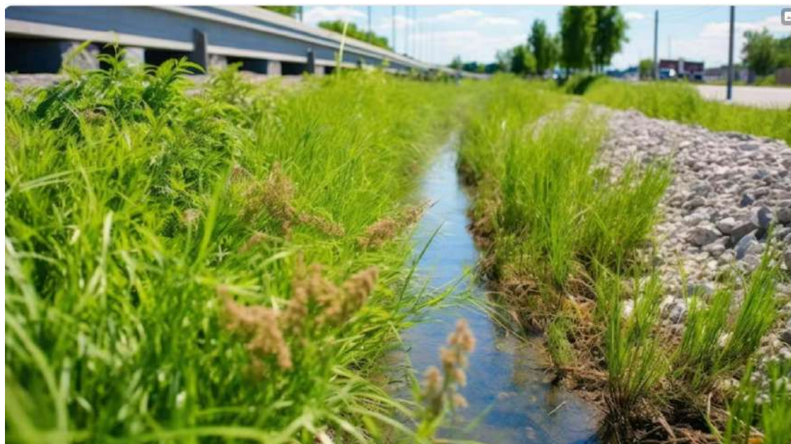
Figure 7-3: A vegetated swale used for a roadside runoff application. Source: www.stormwater.com
