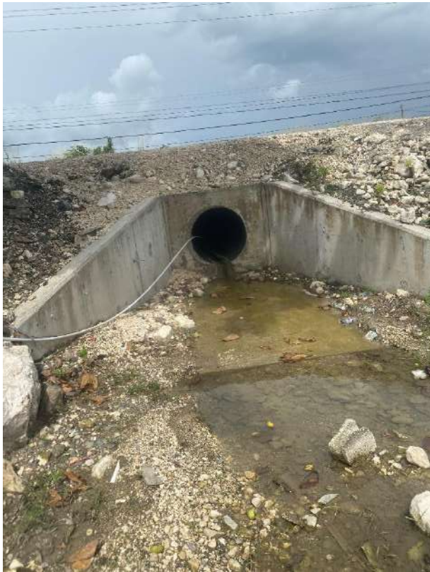
Figure 6-13: An 800mm culvert that crosses the highway and empties in the foreshore
