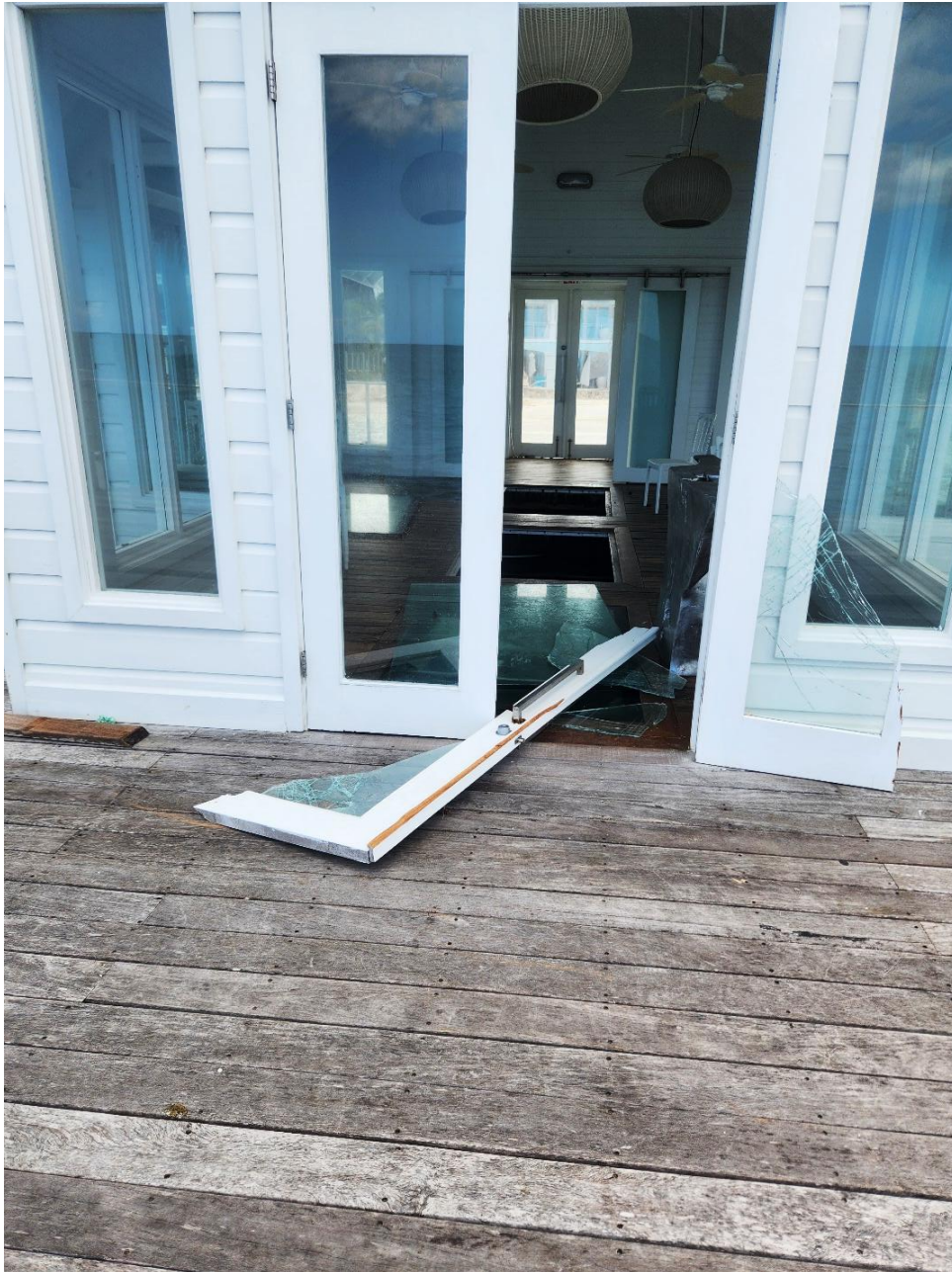
FIGURE 5-51: THE HOUSE OVER THE WOOD PIER (2ND FROM THE EAST) WAS DAMAGED BY THE SEVERE WINTER STORM IMPACTED JAMAICA ON FEBRUARY 6, 2024. THE GLASS BOTTOM WAS DETACHED BY THE WAVE IMPACT FROM UNDERNEATH. THE DECK IS ROUGHLY 1.3 M FROM MEAN SEA LEVEL. PHOTO WAS TAKEN FEBRUARY 11, 2024 ABOUT 5 DAYS AFTER THE STORM.
