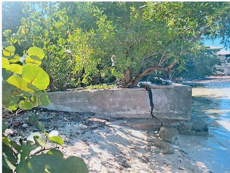
Plate 42: A tree was observed growing through the concrete, causing it to crack
