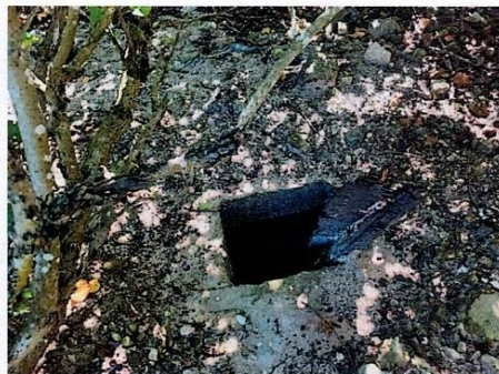
Plate 38: An exposed manhole
