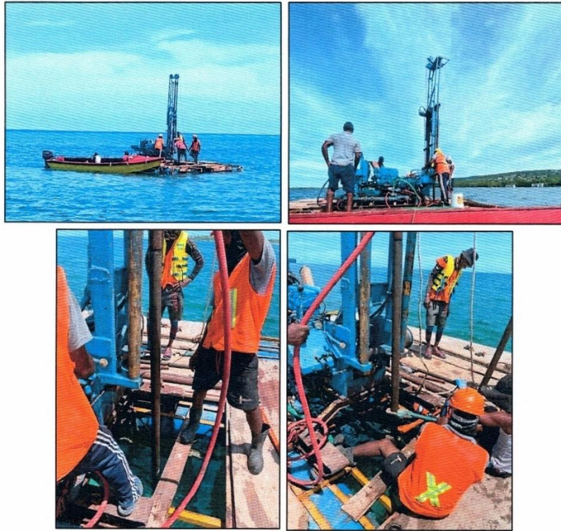
Plate 3-1: Offshore borehole drilling at Sandals, Montego Bay using a Barge mounted Drill Rig
