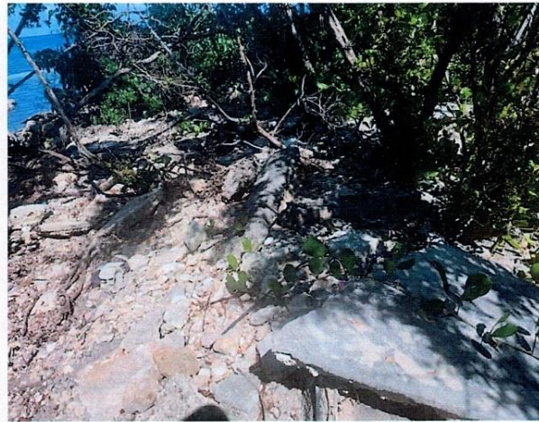
Plate 20: Uplifted concrete foundation
