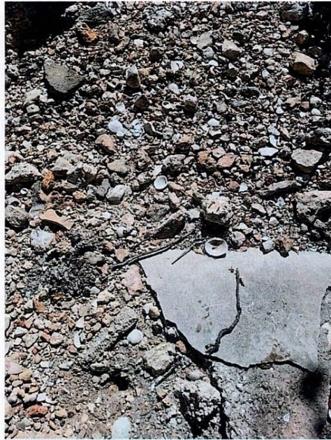
Plate 19: Displaced concrete foundations
