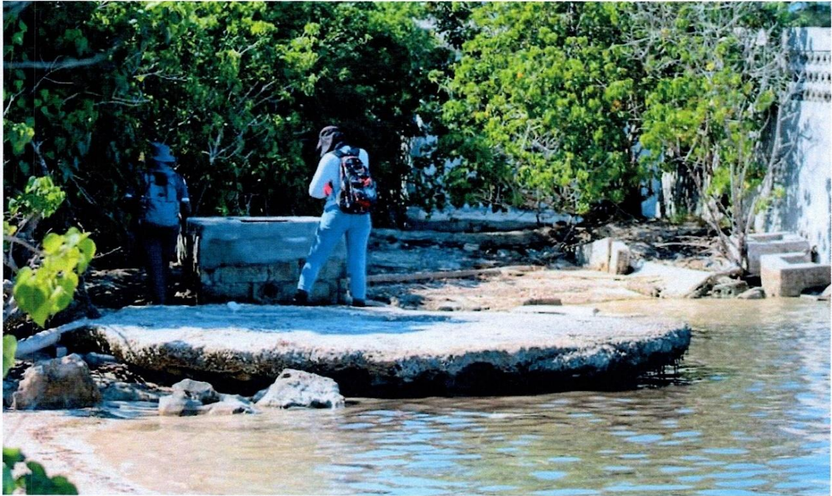
Plate 37: Uplifted concrete foundation with cistern nearby
