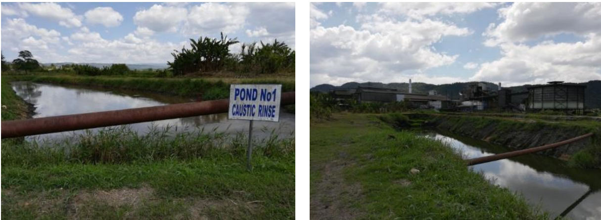
Picture 23 - Appleton estate wastewater treatment component (source: SCP)
