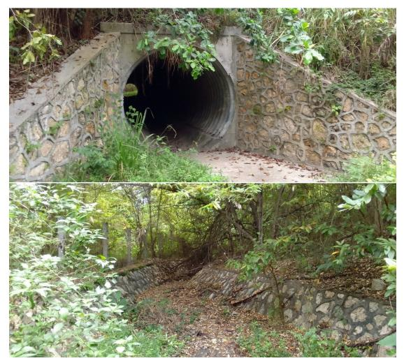
Figure 4-37: Drainage system from the western to eastern sides of Edward Seaga Highway (North/South Highway). Upper photograph shows drain channel under the highway; lower photograph shows small canal on the western side of the highway leading southwards to the area (Conolley photo 2022)
