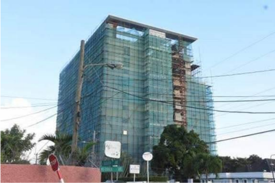
Plate 11G 52 : Construction Containment Nylon Mesh Deployed Around a Construction Site In Kingston.
