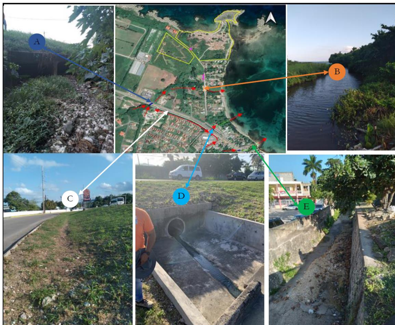
Figure 5-22 Existing drainage features within the catchment area showing (A) Double Box Culvert, (B) Earth Drain that discharge into the sea, (C) earth swale, (D) Pipe Culvert and (E) Open U Channel
