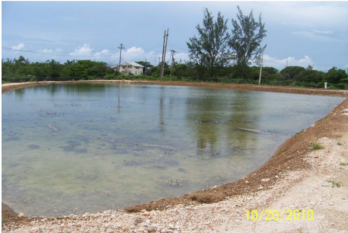
Plate 7 Photo flooded treatment area of landfarm
