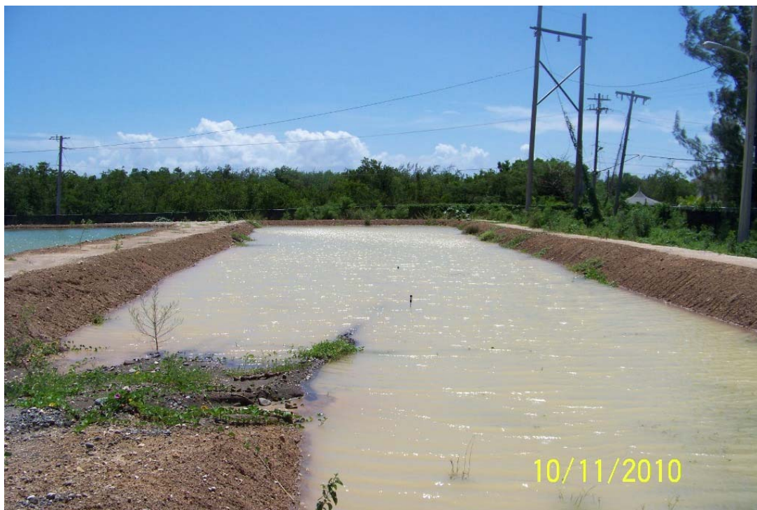
Plate 6 Photo showing flooded storage area of landfarm
