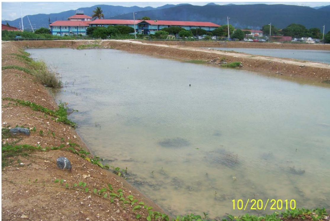
Plate 10 Photo showing flooded storage area at landfarm
