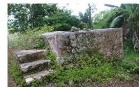
Cut stone water tank
