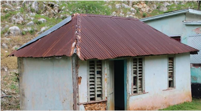
Plate 90: Vacant vernacular house with nog walling, jalousie windows and hip roof
