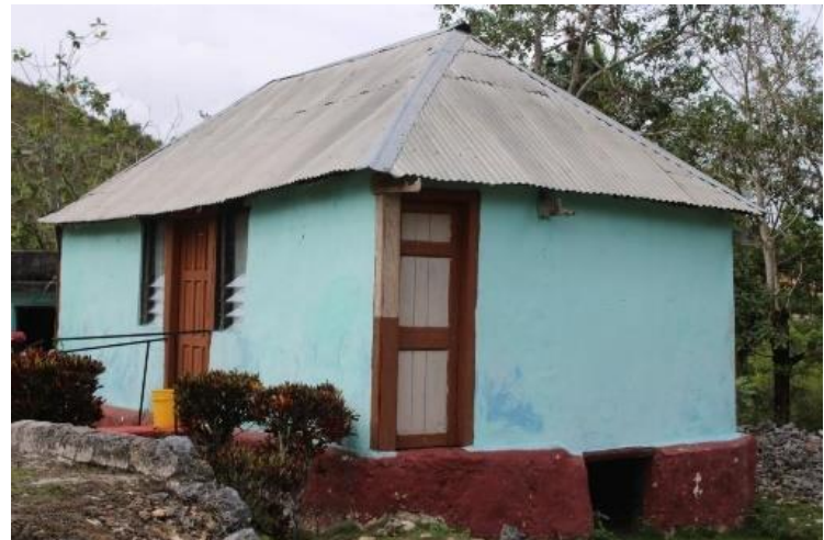
Plate 121: Small well maintained nog house with hip roof and brown cut stone foundation
