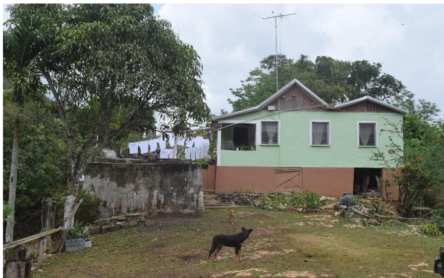
Plate 172: Plate Large vernacular nog-wall house and square cut stone water tank in Camperdown, St. Ann.
