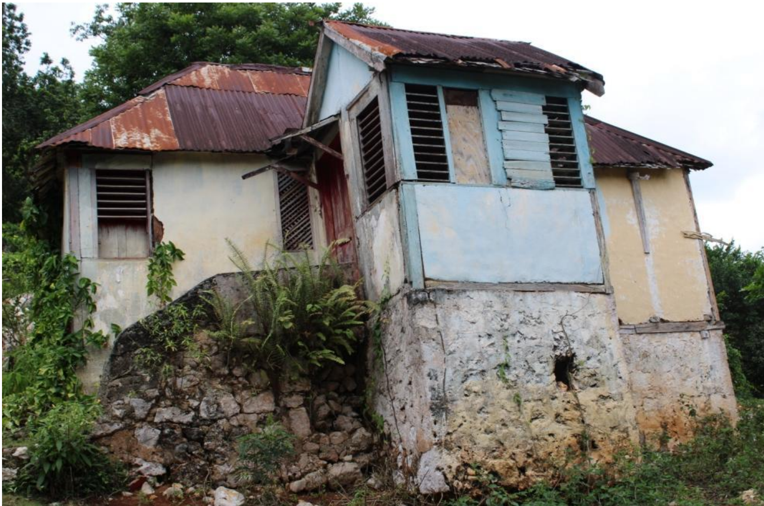
Plate 128: Vernacular house on a hill with a high cut stone foundation and hip and gable roof. Historical graves, a water tank and a barbecue are also present
