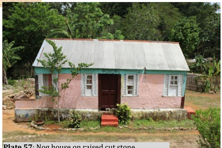
Plate 57: Nog house on raised cut stone foundation with a gable roof. (Lincoln, St. Ann)
