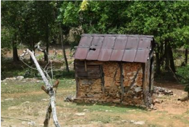
Plate 108: Detached degenerated nog wall kitchen with zinc gable roof.
