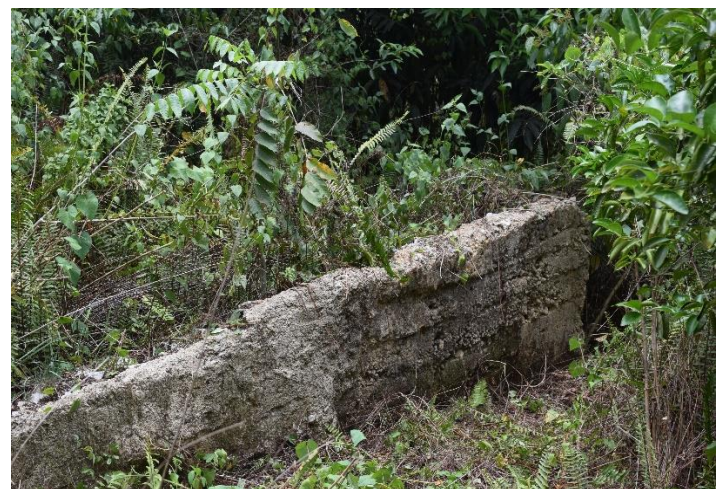
Plate 40: Stone foundation rendered with lime mortar
