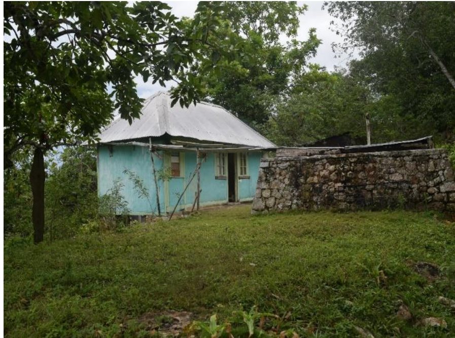
Plate 173: Small nog house on raised cut stone foundation beside square cut stone water tank. (Camperdown, St. Ann)
