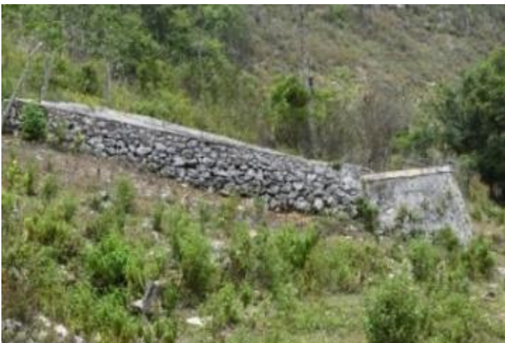
Plate 110: Circular cut stone water tank with elevated catchment.
