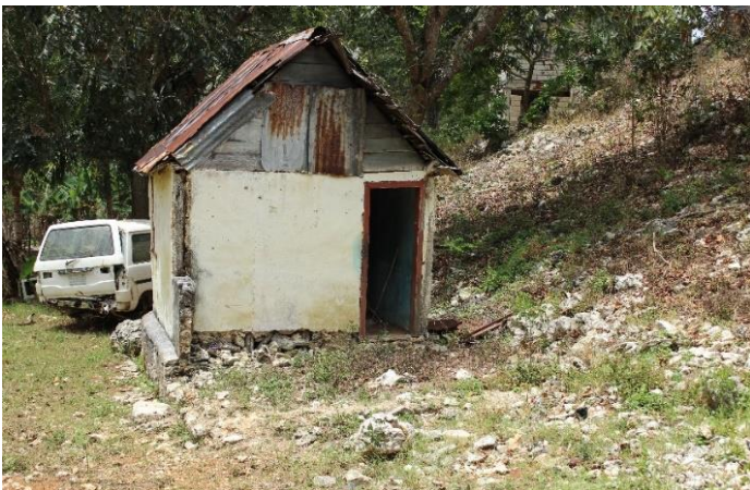
Plate 60: Small nog wall house on raised cut stone foundation. (Lincoln, St. Ann)
