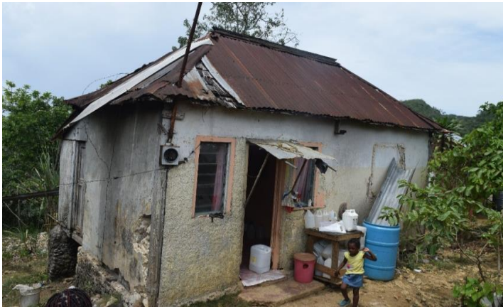
Plate 135: Small nog-wall house on raised cut stone foundation with small cellar and square water tank. (Clover Hill, St. Ann)
