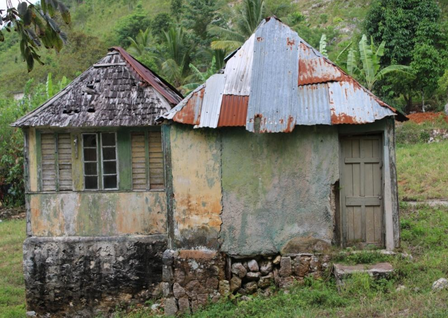
Plate 79: Side view of abandoned vernacular house with hip roofing, french and jalousie windows and cut stone foundation
