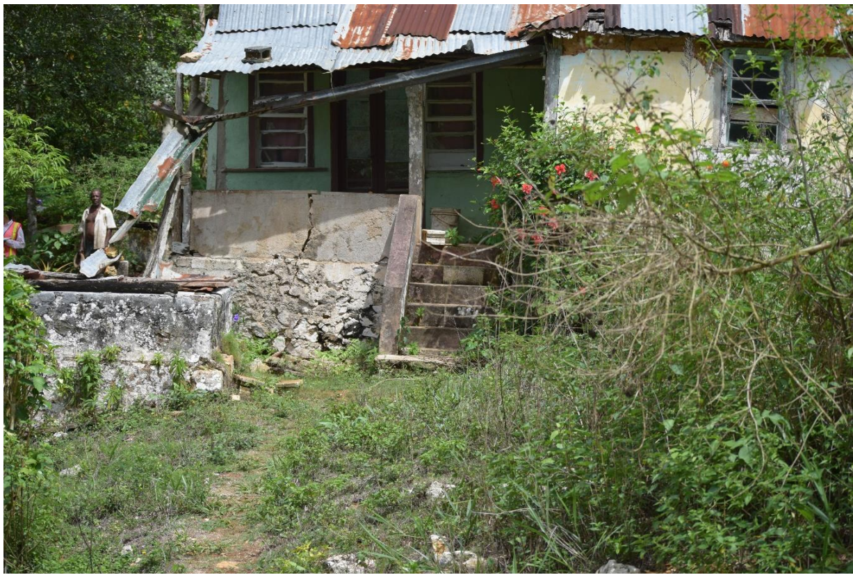
Plate 184: Extant, degenerated nog-wall house on raised cut stone foundation with zinc hip roof showing exposed original wooden shingles underneath. (New Hall, St. Ann)
