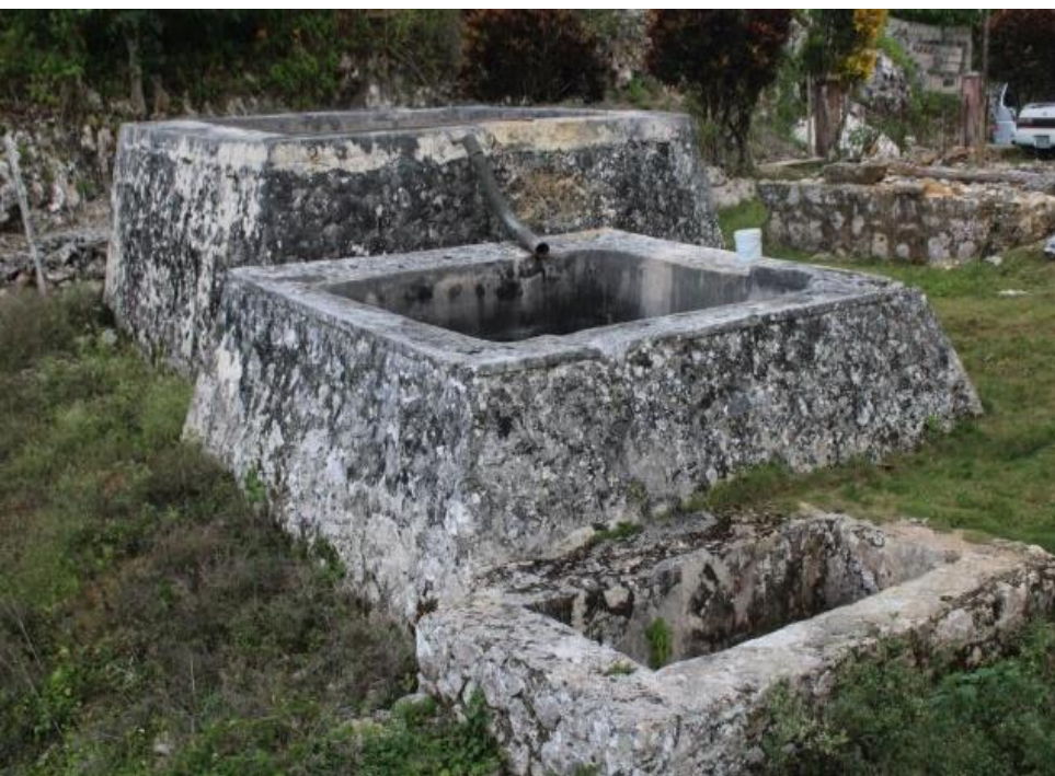
Plate 30: Extant three part cut stone water tank system
