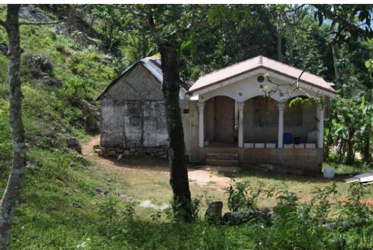
Plate 43: Nog wall house with concrete additions with small family plot with three historical graves made from cut stone and nog material
