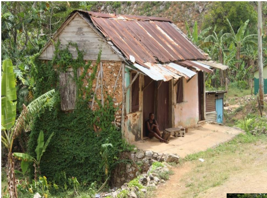
Plate 56: Nog wall shop with gable and pitch roof (original wooden shingles exposed) built atop raised cut stone foundation. (Lincoln, St. Ann)
