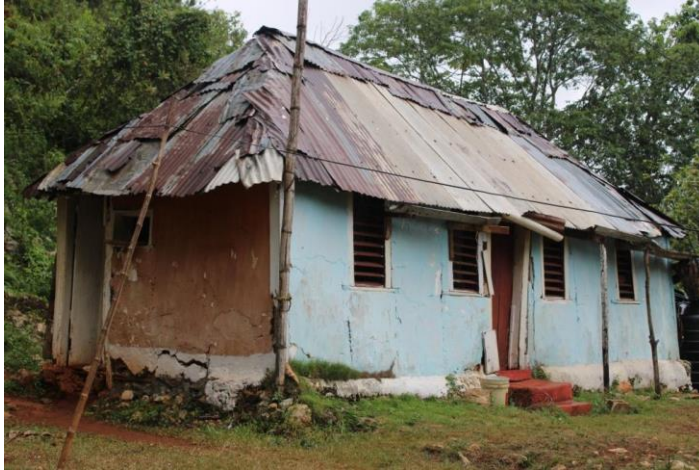
Plate 118: Vernacular house with hip roof and jalousie windows, cut stone foundation and red steps
