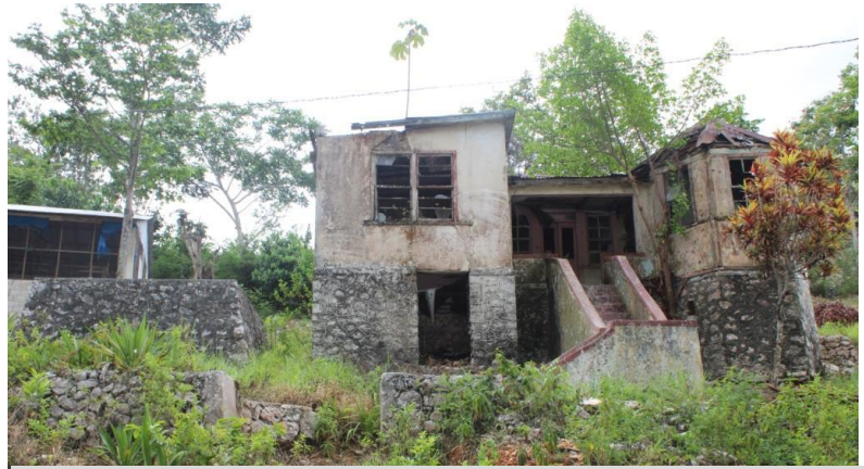
Plate 91: Dilapidated vernacular house with high cut stone foundation, double swing doors and partial hip roof
