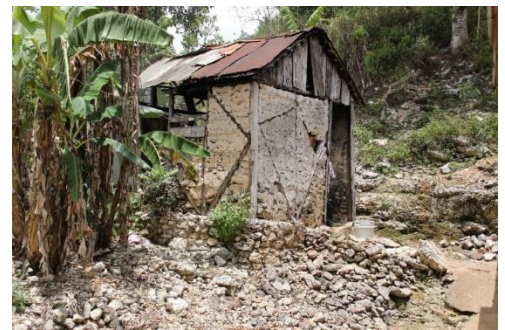
Plate 59: Small extant, dilapidated nog wall kitchen at the back of a modern house
