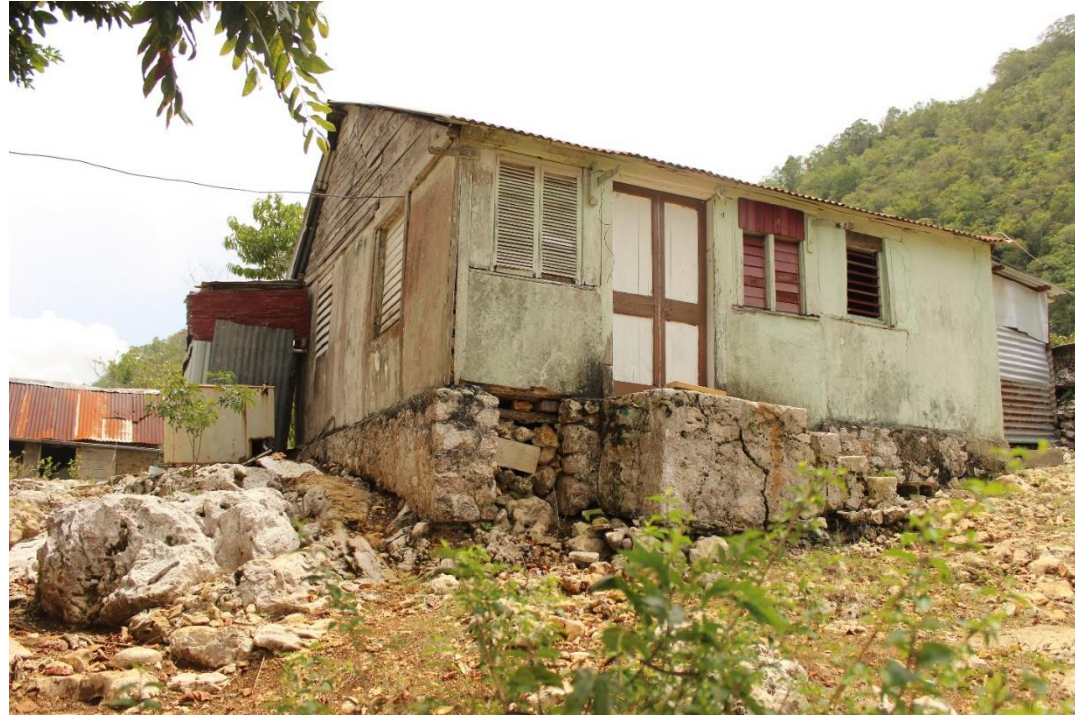
Plate 175: Small nog-wall house on raised cut stone foundation in St. Johns, St. Ann.
