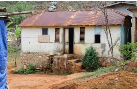
Plate 120: Vernacular house with jalousie windows and cut stone foundation with cellar, cut stone tank in yard
