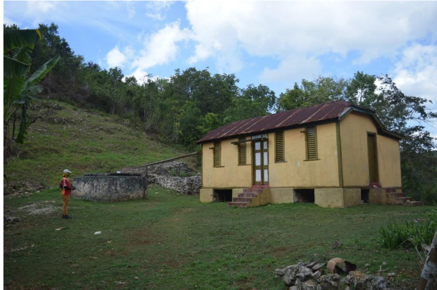
Plates 186 and 187: Nog house on raised stone stilts, painted cream.
