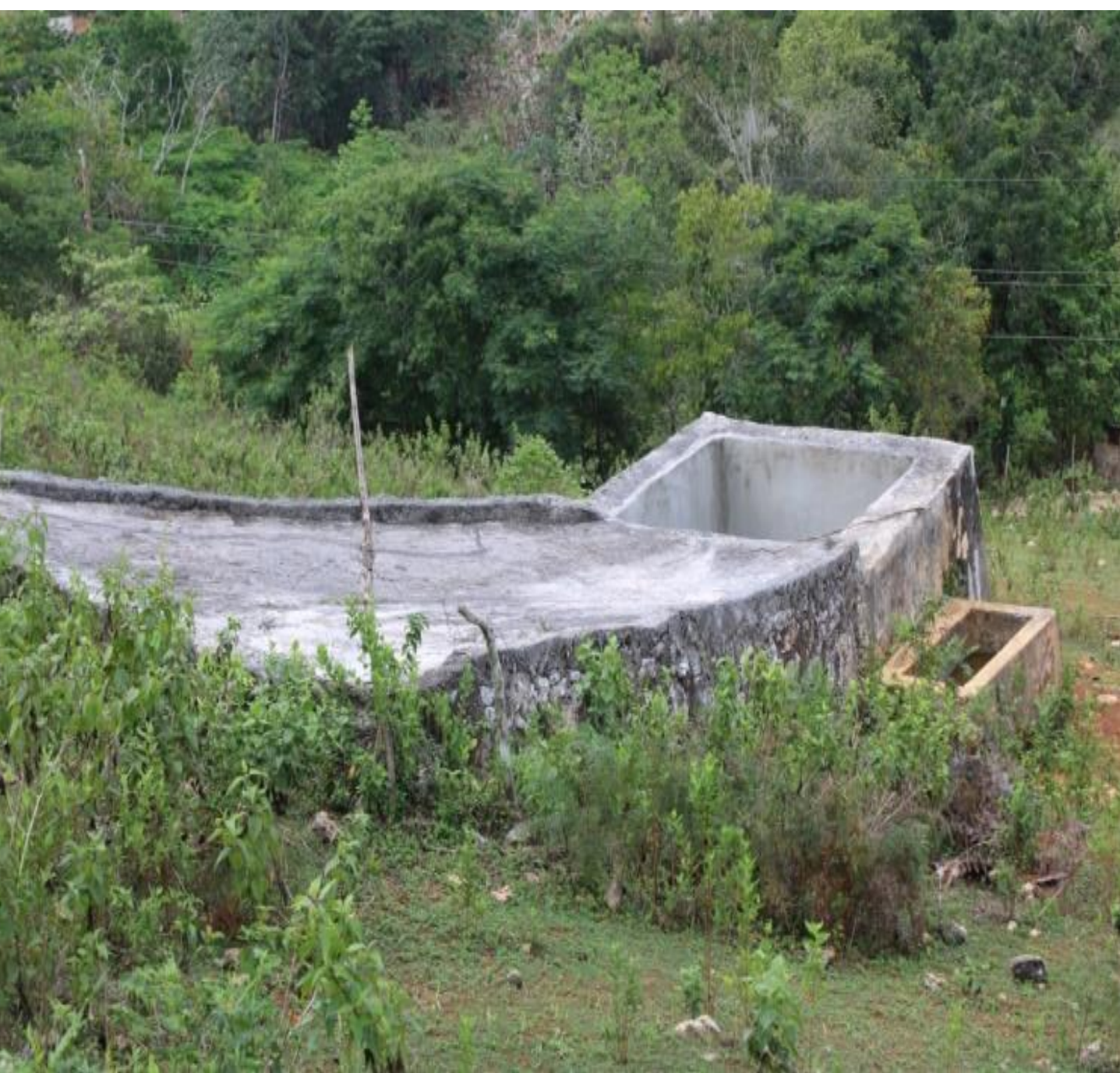
Plate 170: Cut stone water tank with a long narrow catchment
