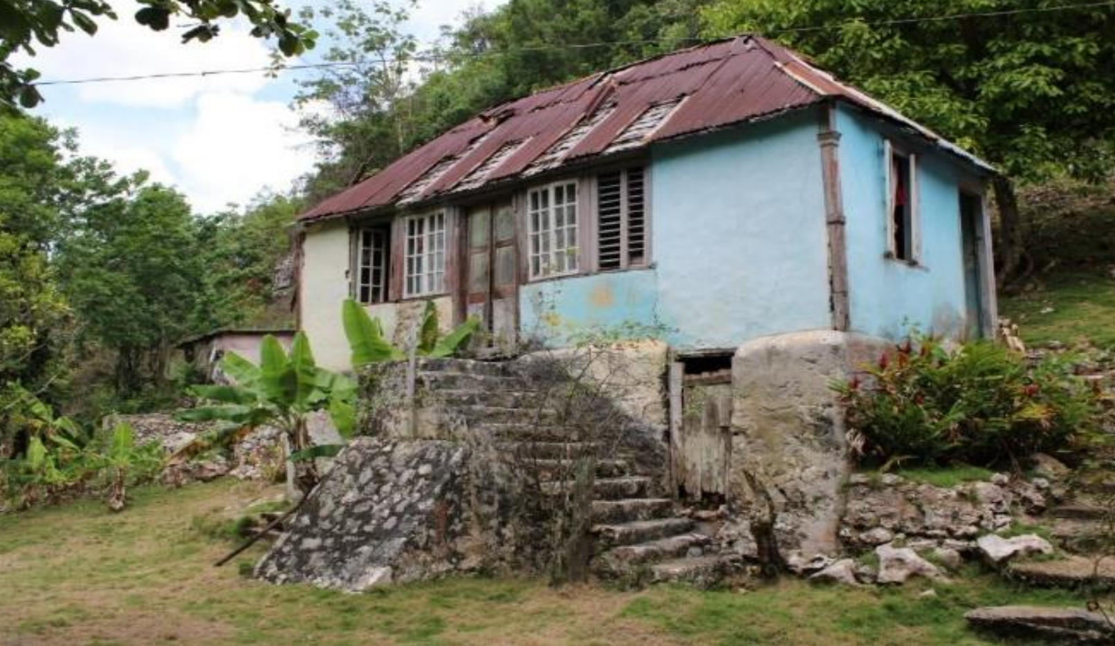
Plate 126: Blue vernacular house with hip roof which has shingle under the zinc. It has sash and jalousie windows and stone steps.
