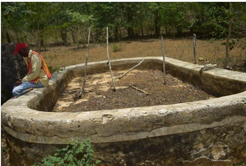
Plate 104: Unusually shaped water tanks elliptical in shape located in depressions on lands used as cow pastures.
