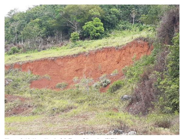
Figure 8-13: Near Vertical Collapsed Bauxite Cliff Face
