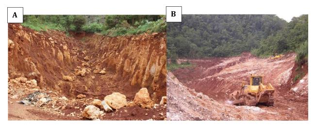
Figure 8-1: [A] Appearance of a typical mined out orebody | [B] Backfilling in progress using three bulldozers to re-profile mined out orebody by cutting and pushing material from higher margins into the main depression.
