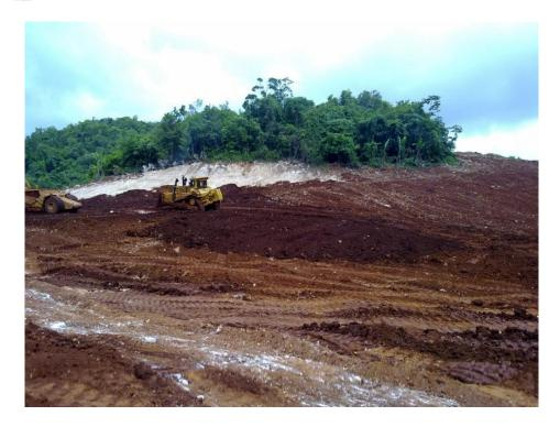
Figure 8-4: Topsoil spreading in progress using scraper and bulldozer
