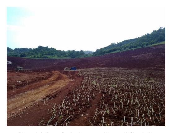
Figure 8-6: Grass planting in progress in topsoiled orebody
