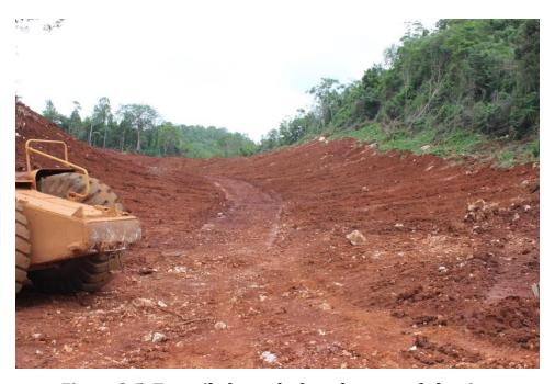
Figure 8-5: Topsoiled area before the start of planting
