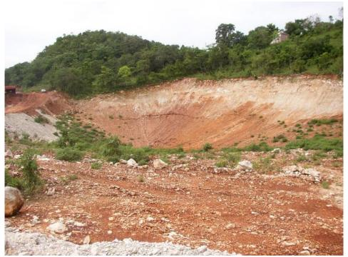
Figure 8-2: A reshaped orebody before start of topsoiling process
