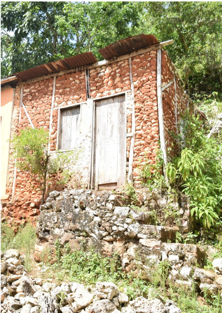
Plate 2: A recently constructed nog wall house using wood from the forest as supporting frame and fabrication of doors and windows. The structure was built on the foundation of a similar type of historical house. The stone steps and foundation are testimony to the former historical structure.
