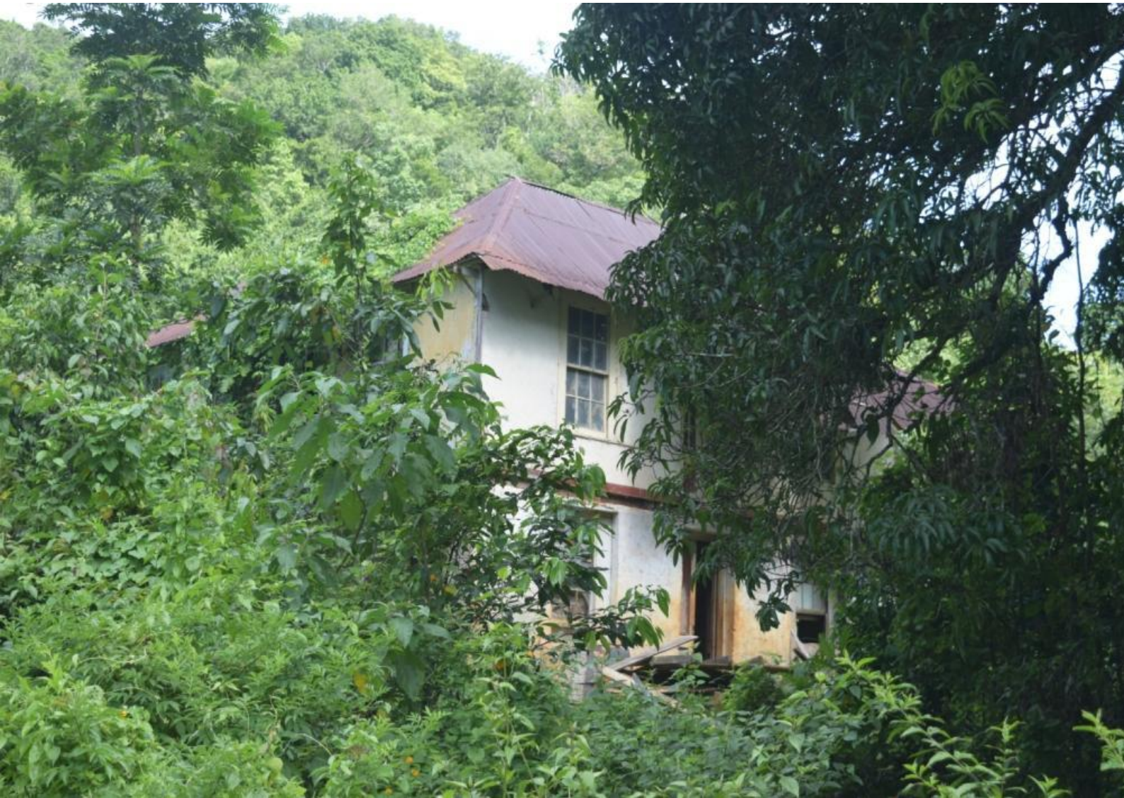
Plate 31: The Belmont House, a two storey cutstone and nog wall structure with sash windows and hip roof.
