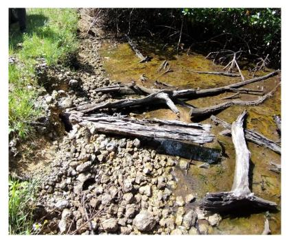
Figure 1.12: Western access road with log beneath roadway provides visible route for freshwater movement below the road
