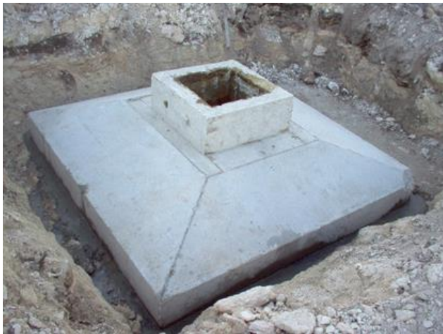
Plate 5-2 Candlestick footing placed inside excavation
