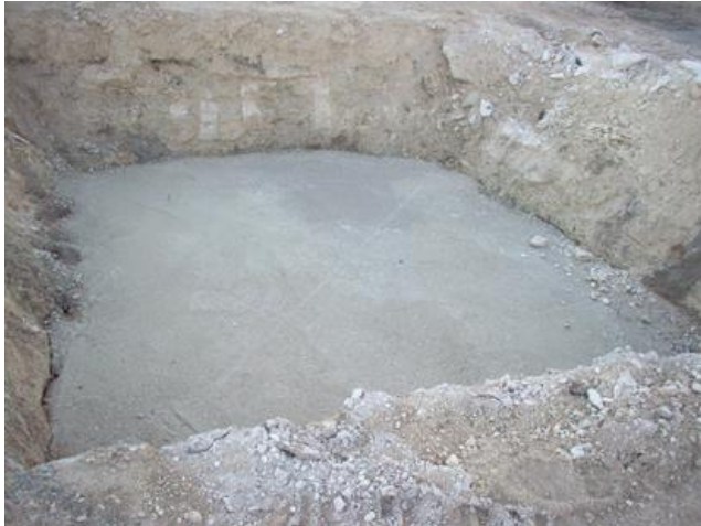
Plate 5-1 Concrete poured into excavation
