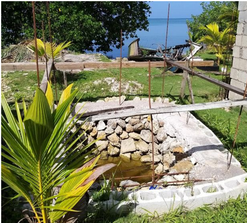
Plate 6-65 Soakaway pit under construction at a property west of proposed hotel project property
