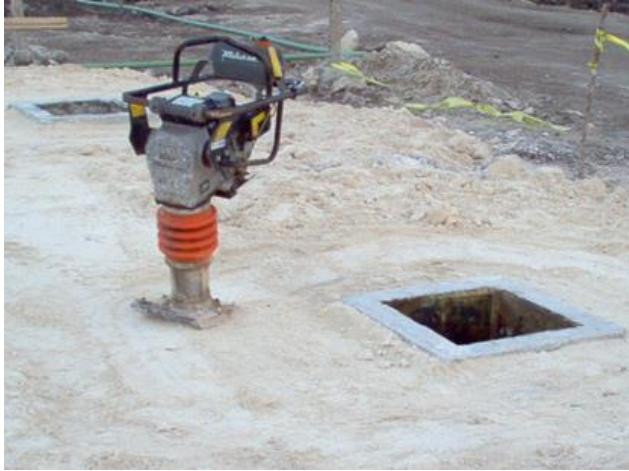
Plate 5-3 Filling of stump and compaction
