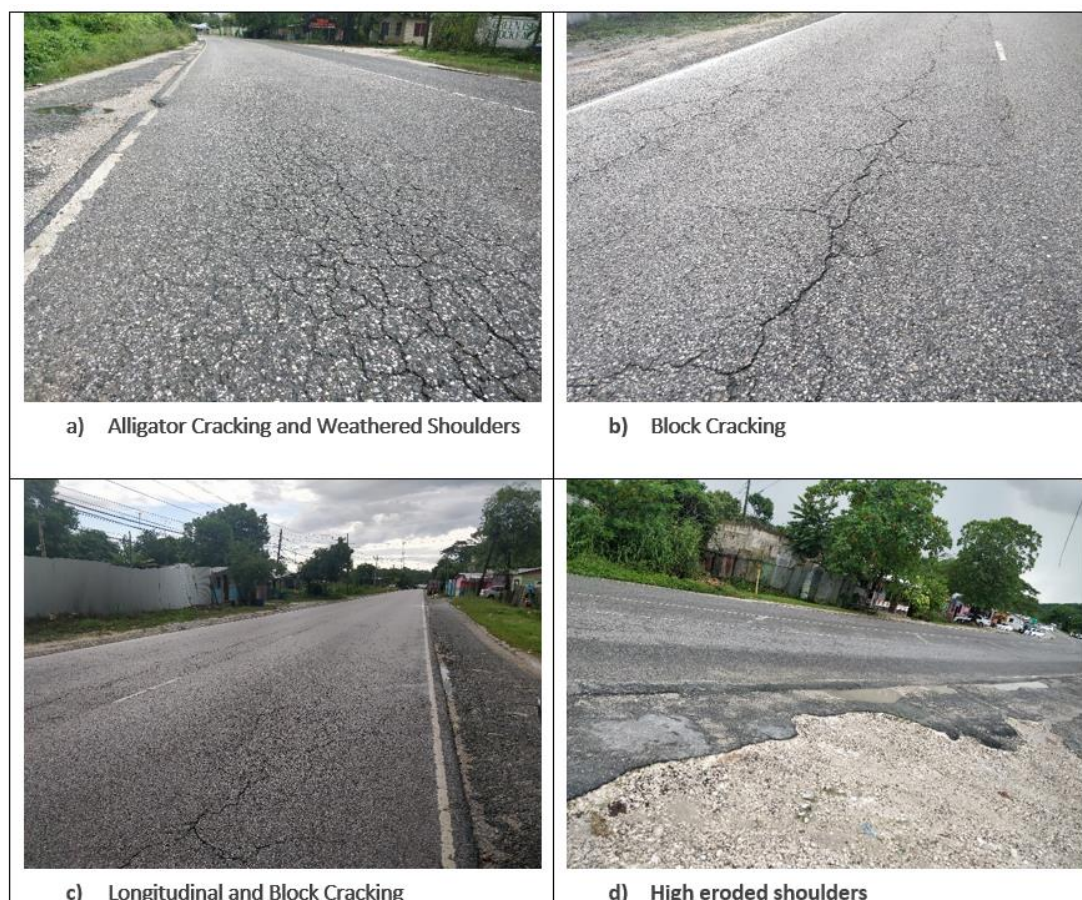
Plate 6-67 Distresses identified along the road surface
