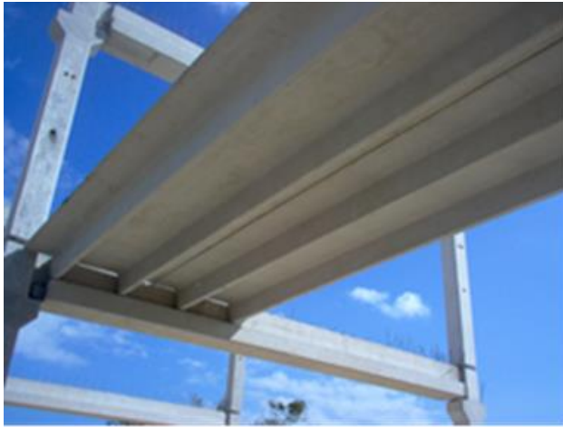
Plate 5-5 Beams placed atop columns
