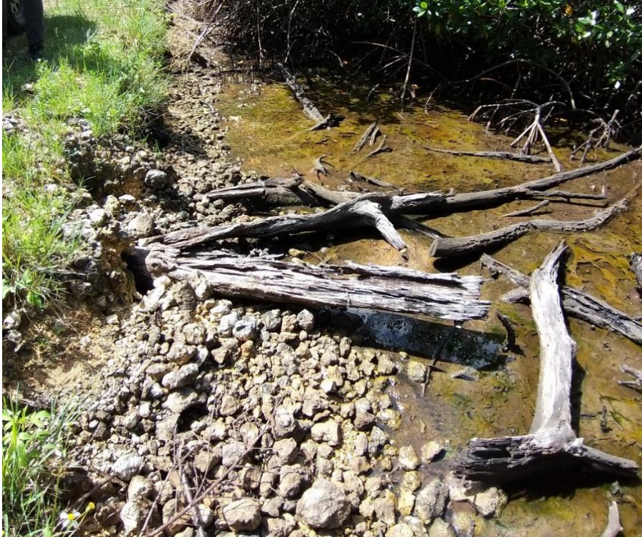
Plate 6-2 Western access road with log beneath roadway provides visible route for freshwater movement below the road
