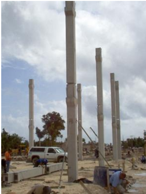
Plate 5-4 Columns placed in candlestick footings
