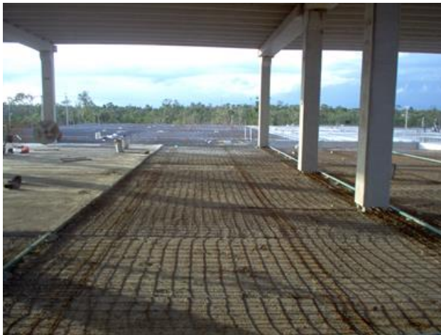
Plate 5-6 Reinforcement of areas using electro welded mesh
