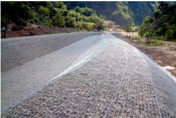
Plate 5-13 Reno Mattress installed along River
