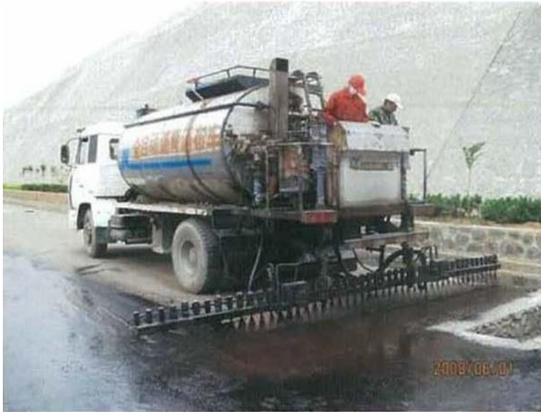
Plate 2-1 Asphalt Pavement Construction (Spraying)
