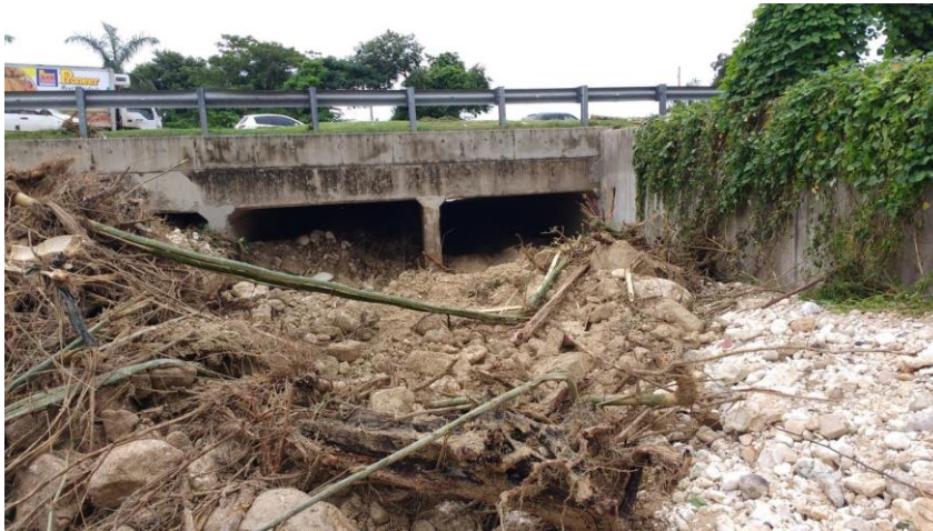
Plate 3-28 Photo of Salt Spring Gully, significantly blocked by debris and sediments (Assessment of the St. James November 2017 Flooding, 2018)
