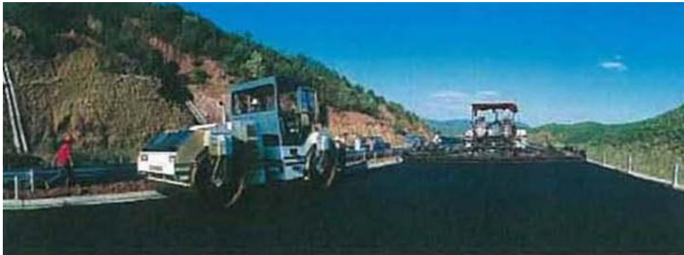
Plate 2-4 Spreading and Compacting Asphalt Mixture
