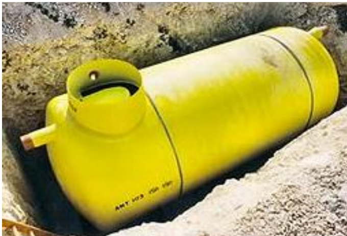
Plate 5-16- Filling station forecourt separator
