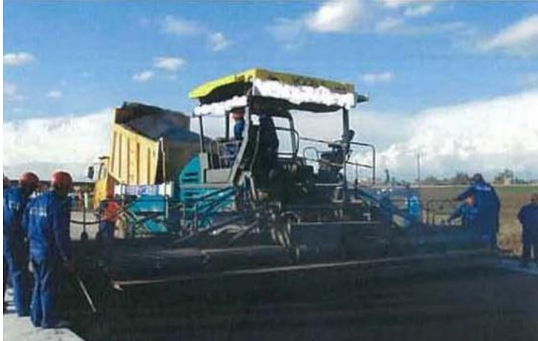
Plate 2-3 Asphalt Concrete Spreading
