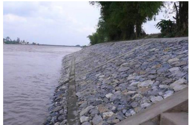
Plate 5-14 Revetment installed along banks of river
