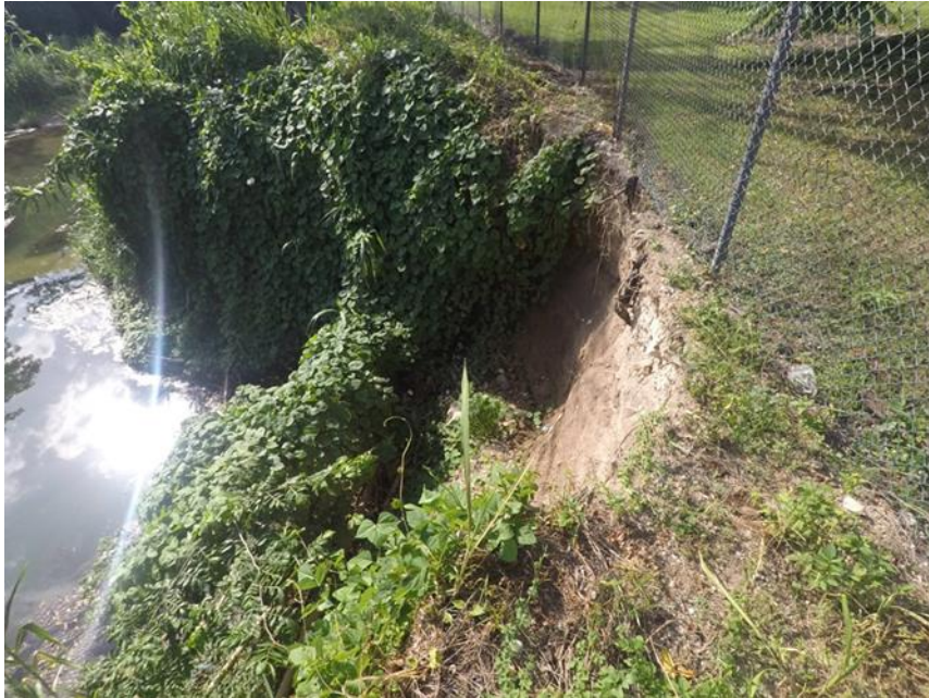
Plate 3-8 Undercutting of the right bank of the Montego River near milepost # 173+700
