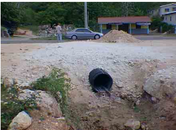
Figure 8 Culvert downstream of road at Location 3
