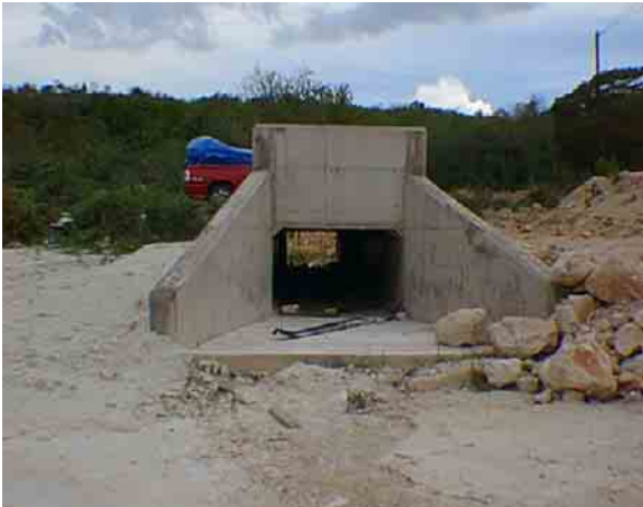
Figure 6 Culvert downstream of road at Location 1
