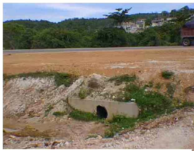
Figure 4 Culvert at location 4
