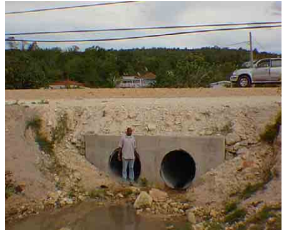
Figure 7 Culvert downstream of road at Location 2
