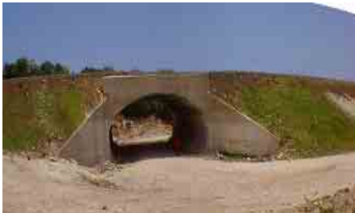
Figure 5 Culvert at Location 5
