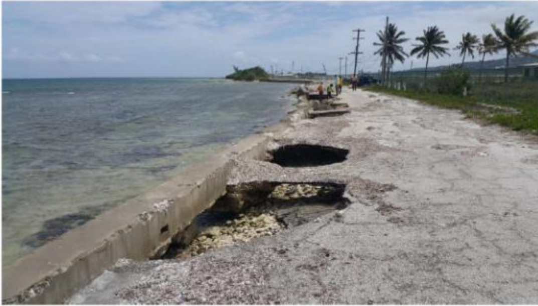
Figure 13: Condition of shoreline protection at the western end of Kent Ave.
