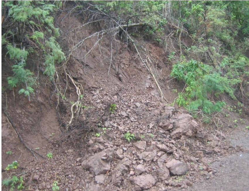
Plate 5.2.3: Landslide on Haul Road near Halberstadt quarry
