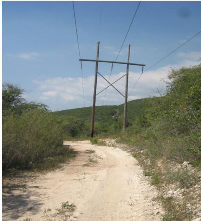
Plate 7.2.1: JPSCo Electrical Transmission Power line located on the south-western boundary of the Harbour Head site.
