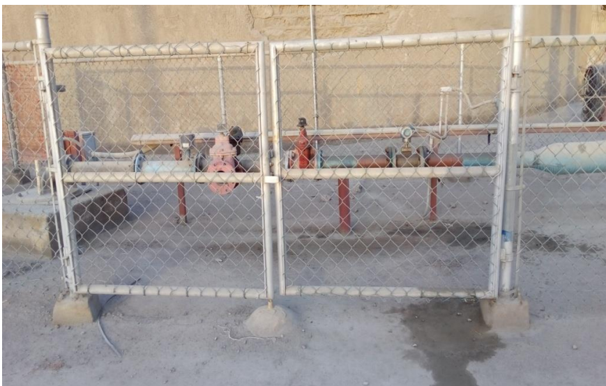
Plate 5.1.16: Well located on the Caribbean Cement Company Plant Site
