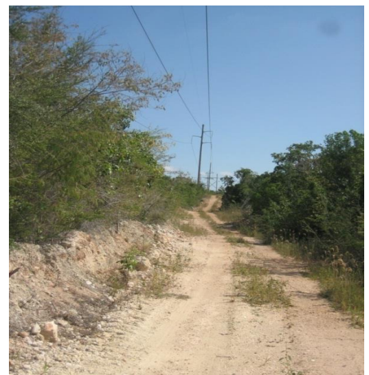
Plate 4.1.1: Access road for JPSCo Electrical Transmission Tower lines used to access
