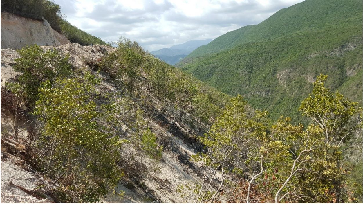
Plate 4.1.6: Existing conditions at Harbour Head
