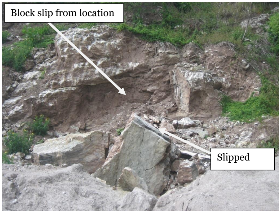
Plate 5.2.4: Rock block failure at the end of quarry face of Halberstadt quarry
