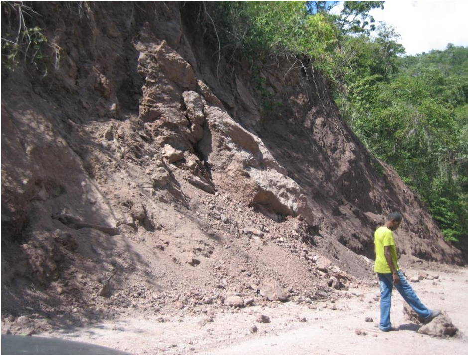
Plate 5.2.5: Large slope failure (rock and debris slide) on main haul road leading into Halberstadt
