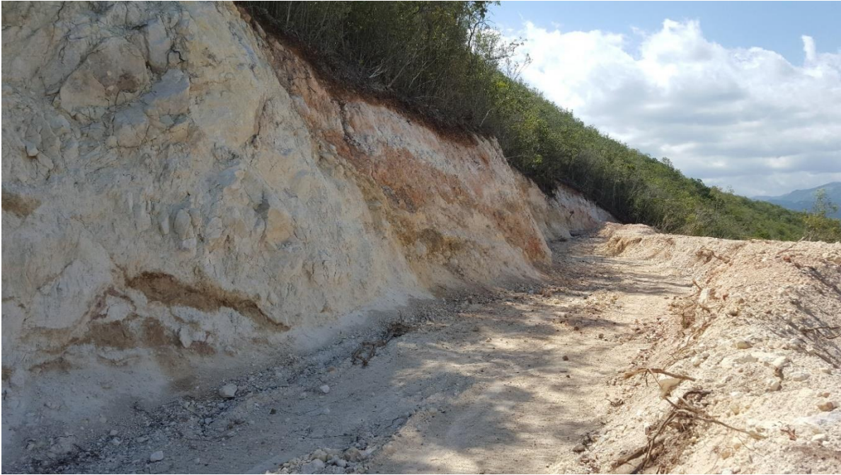
Plate 4.1.8: Existing conditions at Harbour Head
