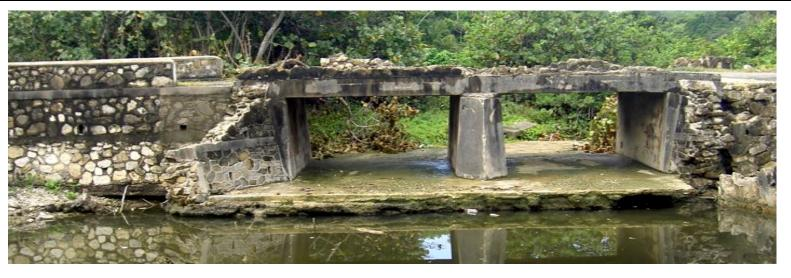
*Figure 20*Box Culvert at the end of the Robins Bay Gully
