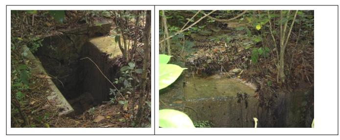
Figure 21Cross Drain Headwall at the source of the Parula Gully
