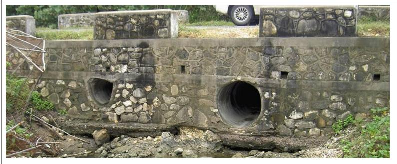
Figure 22 Pipe Culverts at the end of the Parula Gully
