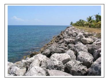
Plate 4.2 Looking NE along stone revetment on north side of headland. This will require the operation of a large excavator at the top of the bank fitted with a hydraulic grapple to individually place and fit boulders on the slope. Constant sorting will be required as smaller boulders are removed from the slope and new ones of proper size are delivered from a nearby quarry.
