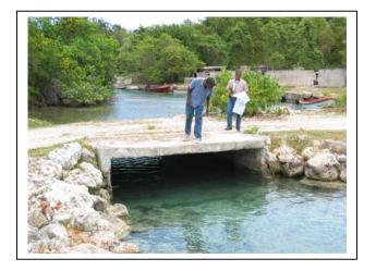
Plate 2.1 Culvert at causeway between mainland and headland at Oracabessa Bay.
