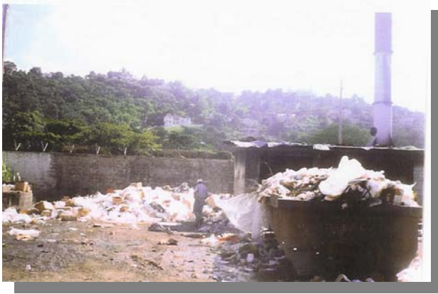
Photo 4.1: Old Disused incinerator.
