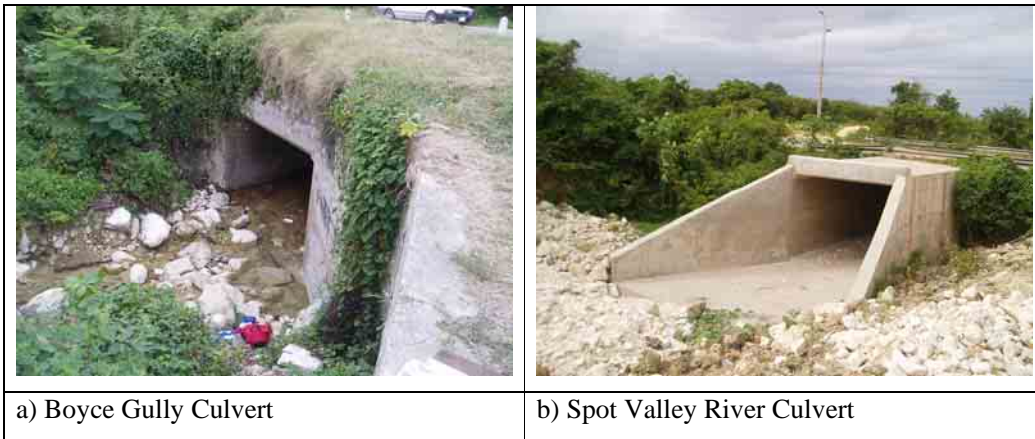
Plate 5.2.5.2 a and b: Box Culverts (viewing on the south side of the road)
