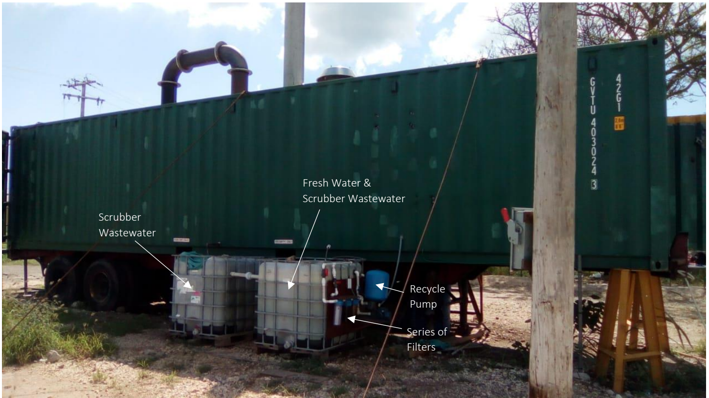
Figure 3.2 Established wastewater recycle system at hazardous waste facility
