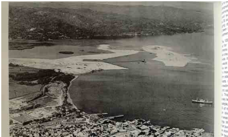
Figure 1.2 Photograph of Montego Freeport - dredging & filling circa 1969. (Source: Jamaica Architect )
