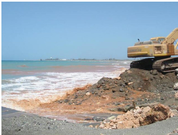
Plate 7-4 Sediment plume from red mud used to pad truck beds to carry armour stone
