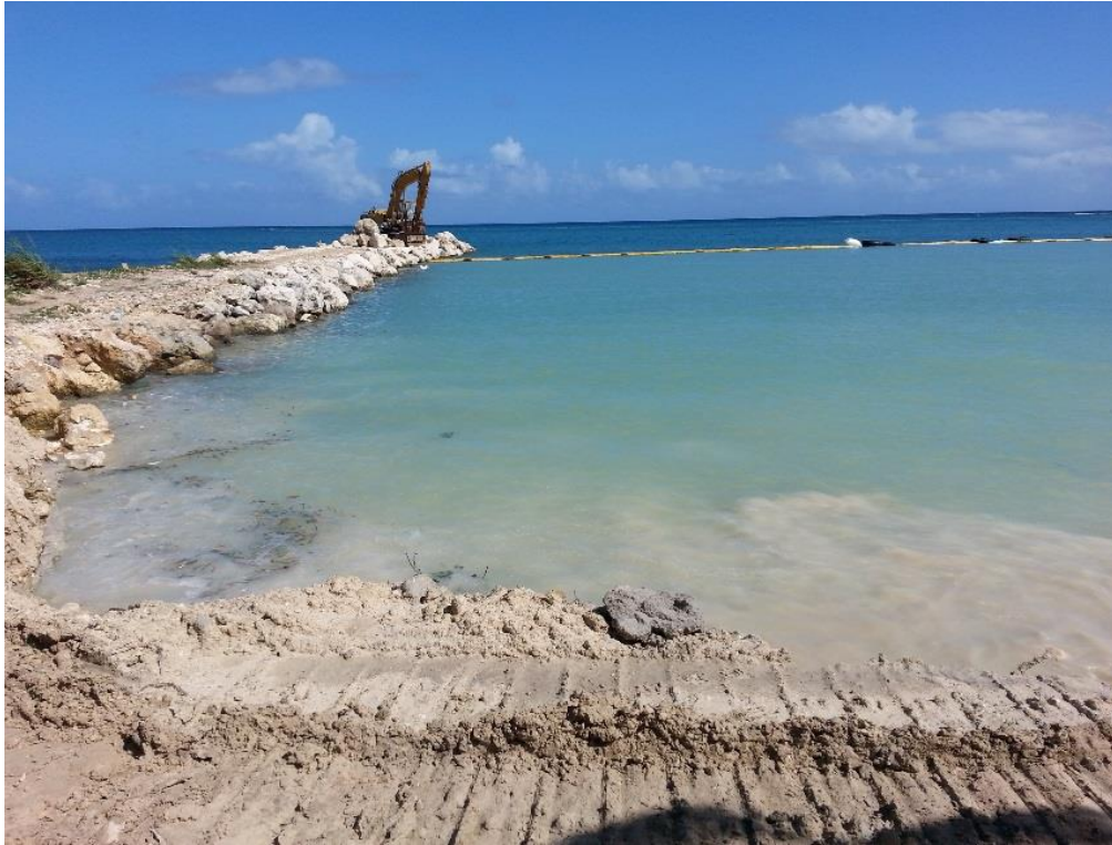
Plate 9-1 Example of a turbidity barrier being used to mitigate against a declining water quality during construction
