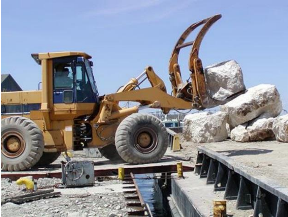
Plate 5-5 Retrieval of boulders using front end loader
