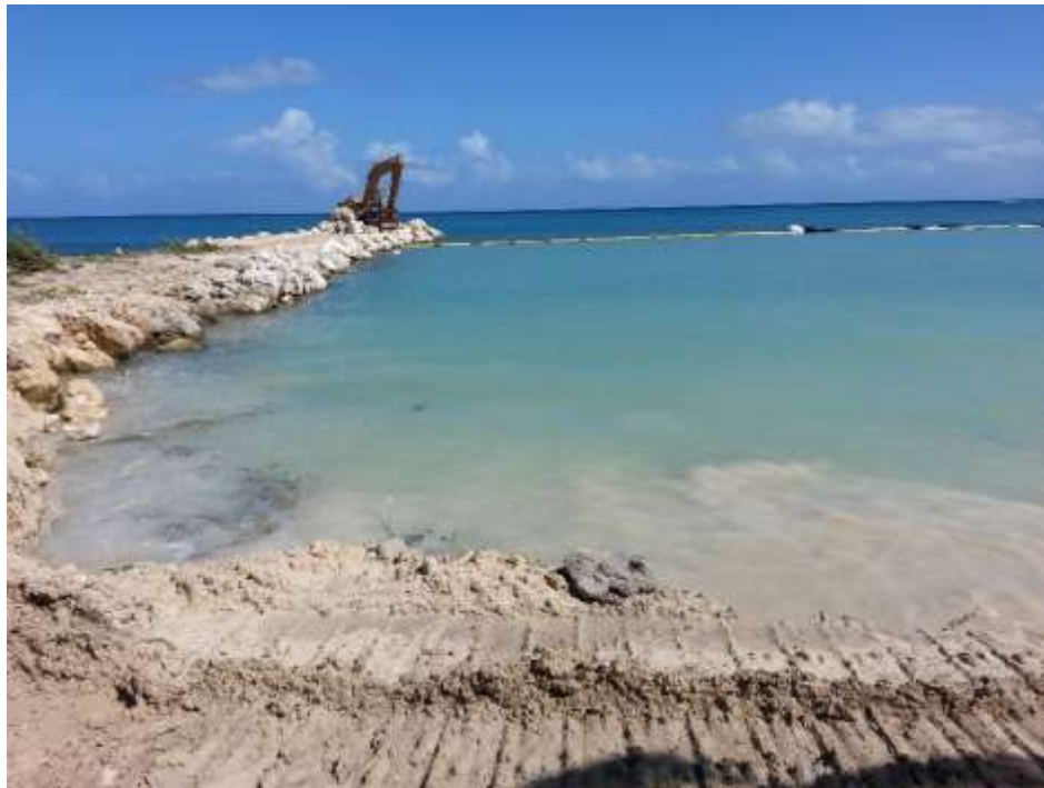
Plate 7-1 Example of a turbidity barrier being used to mitigate against a declining water quality during construction
