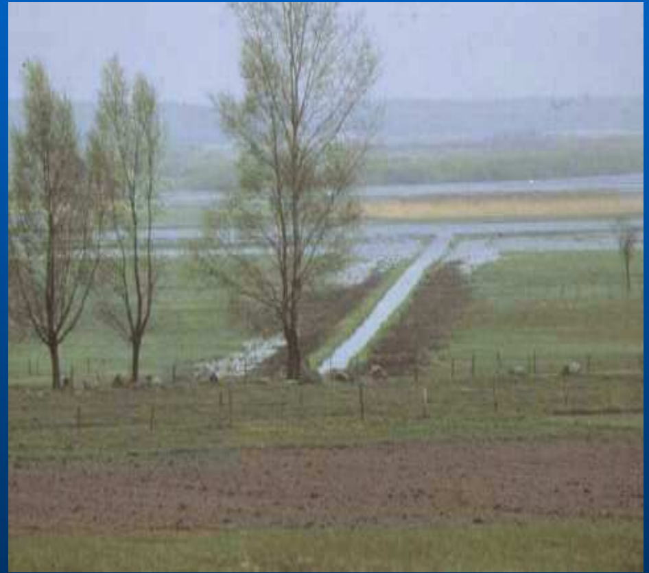
Irrigation canals, Poland
