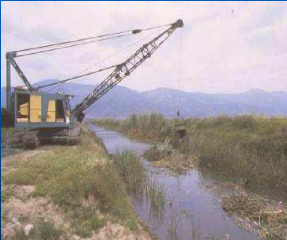
Cleaning of a canal, Turkey
