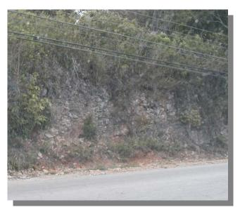
Photo 4.2: Road cut along present main road alignment showing typical characteristics of the main rock type on the site.
