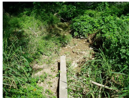
End of culvert just empties onto the ground
