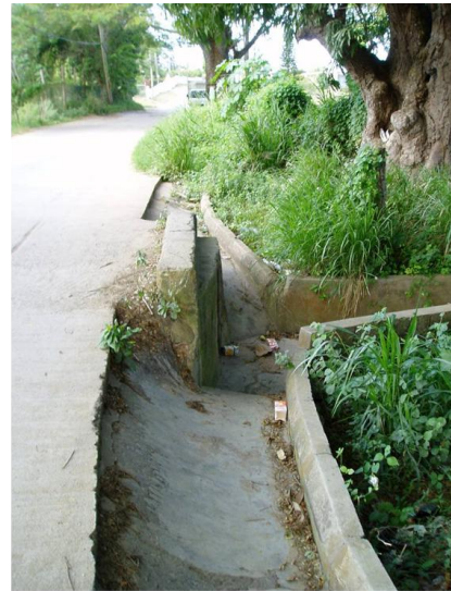
Culvert that now carries runoff under the road from the property
