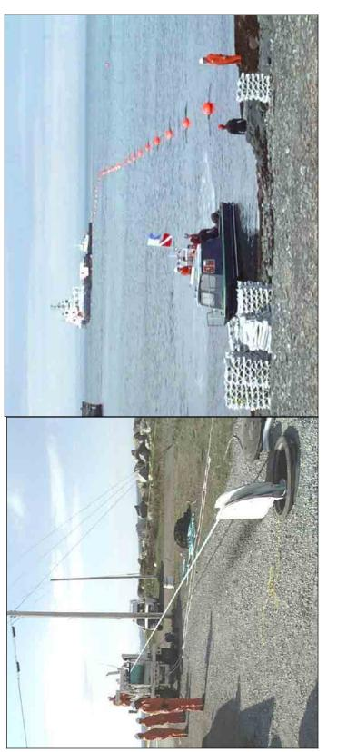
FIGURE 1-19: ILLUSTRATION OF INSTALLATION WITH A WINCH ON THE SHORE; BUOYED CABLE ON THE RIGHT
