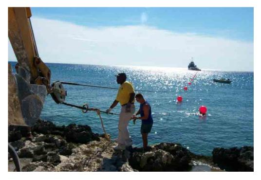
FIGURE 1-18: ILLUSTRATION OF INSTALLATION FROM SHIP WITH A SHEAVE
