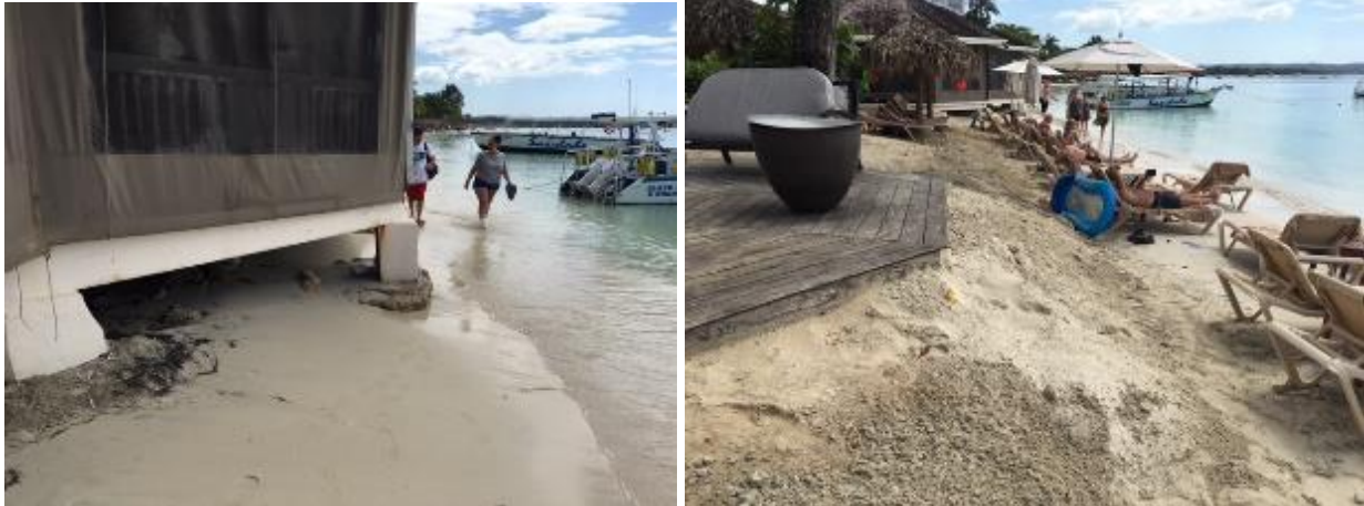
Figure 1-3: Examples of beach erosion occurring at Sandals Negril property (Source: SWIL, 2011)
