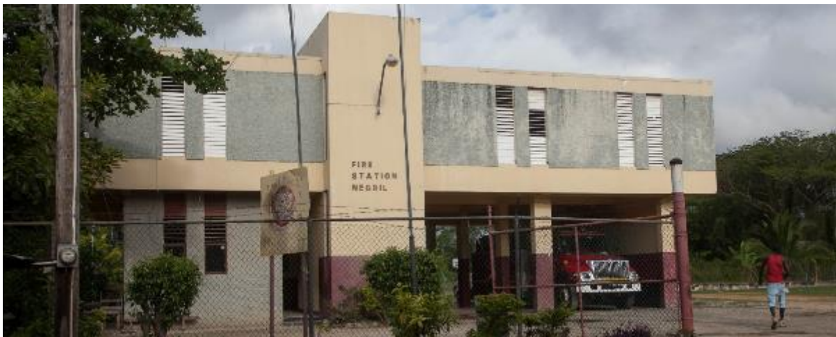
Figure 6-29: The Negril Fire Brigade Station
