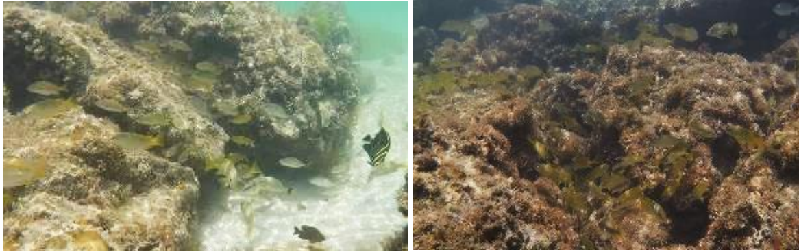
Figure 6-22: Fish foraging within the area of the existing northern groyne (Image source: SWIL, 2018)
