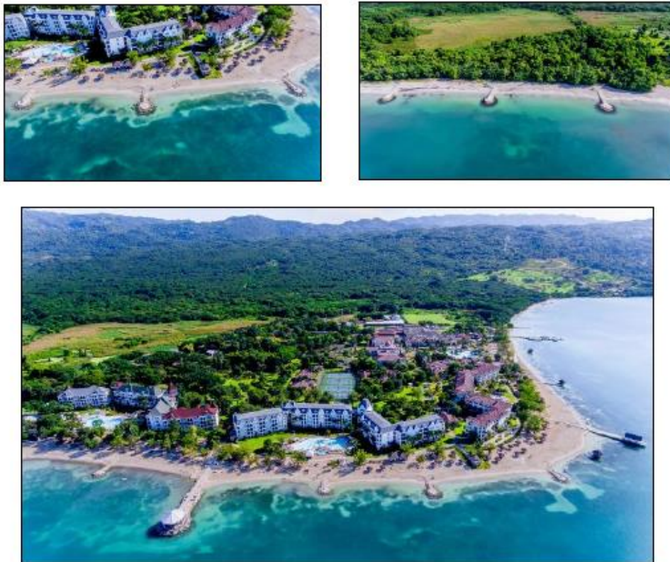
Figure F: Rock groynes at Sandals Whitehouse constructed in 2016-17 to stabilize beach fill amidst a highly eroded shoreline in similar low-energy conditions as Sandals Negril Beach. These groynes are much longer and higher than those proposed at Negril Beach. (The long groyne at lower left was pre-existing prior to the works). Despite highly oblique waves & westerly-directed transport (toward the left in the photographs), little alongshore differential in shoreline location has been observed, and little maintenance has been required.
