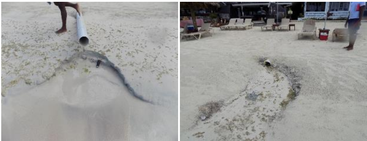
Figure 6-8: Drain pipes emptying into the beach at Sandals Negril
