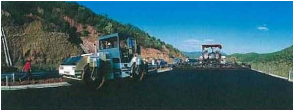
Plate 3-4 Spreading and Compacting Asphalt Mixture (source CHEC)
