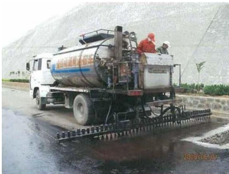
Plate 3-1 Asphalt Pavement Construction (Spraying) (source CHEC)
