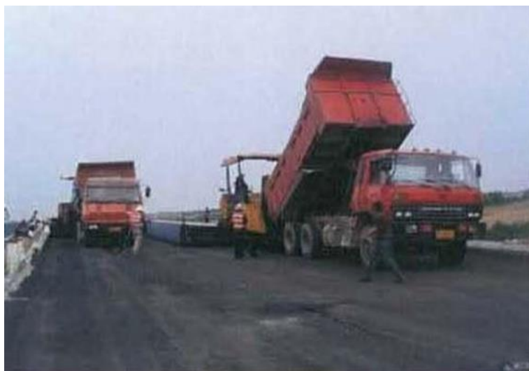
Plate 3-2 Transportation of Asphalt Concrete (source CHEC)
