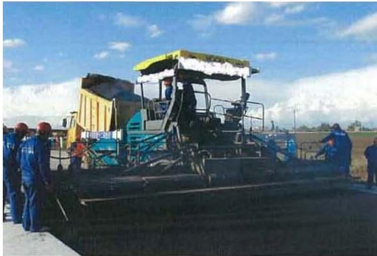
*Plate 2.3 -Asphalt Concrete Spreading (source CHEC)*
