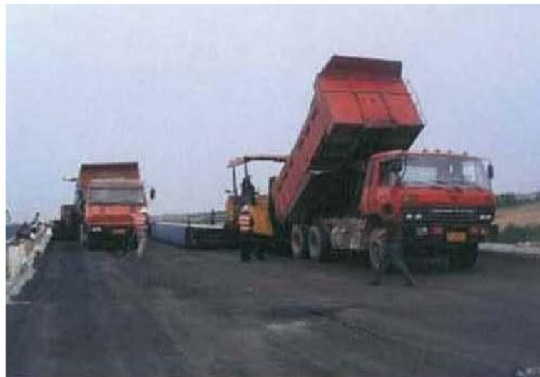
*Plate 2.2 - Transportation of Asphalt Concrete (source CHEC)*
