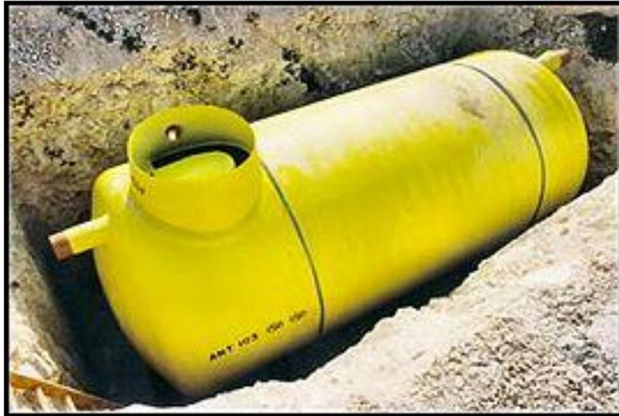
*Plate 9.2- Filling station forecourt separator*
