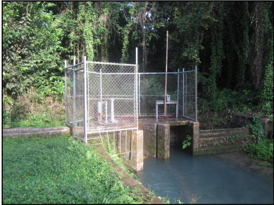
*Plate 4.10 - Sluce gate implemented within the channel of Roaring River*
