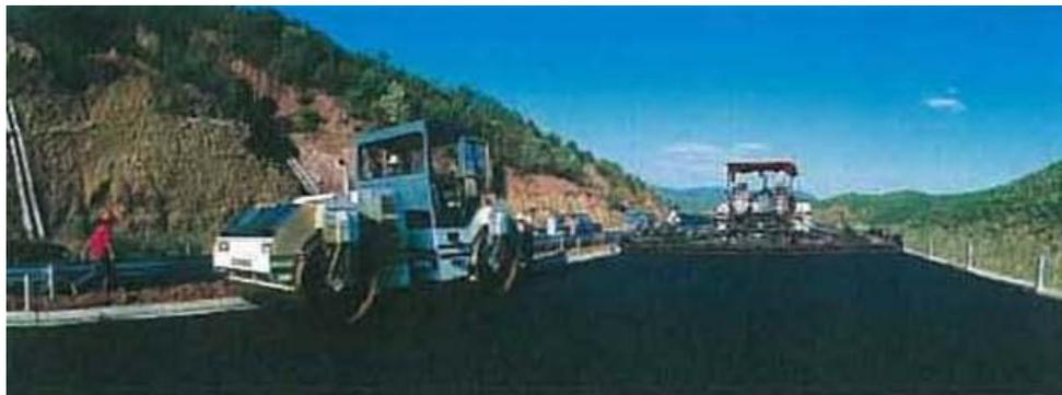
*Plate 2.4 - Spreading and Compacting Asphalt Mixture (source CHEC)*
