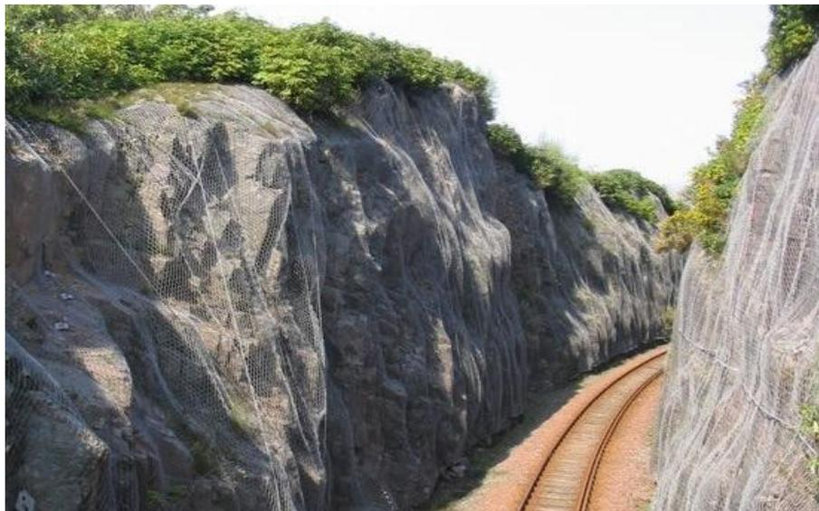
*Plate 9.9 - Rockfall netting used to protect trains from falling rocks*
