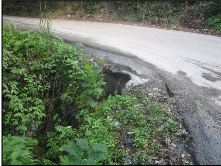
*Plate 4.6 - Exposed culvert pipe under existing roadway*
