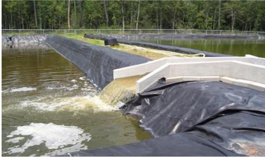
*Plate 9.3 - Detention ponds used to reduce peak flows*
