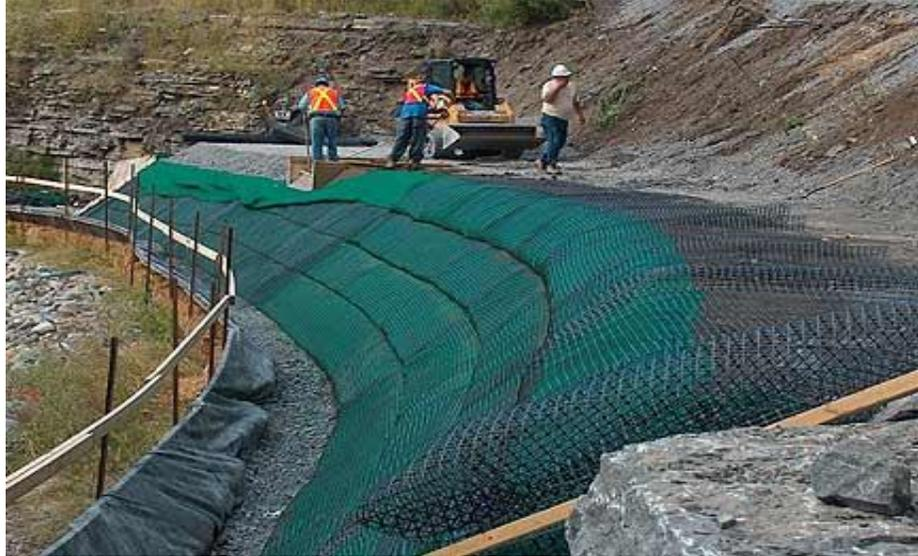
*Plate 9.10 - Geogrids being placed on face of slope*
