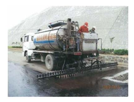
Plate 2.1 - Asphalt Pavement Construction (Spraying) (source CHEC)
