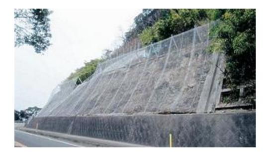
Plate 9.1 - Rockfall catchment fences being implemented
