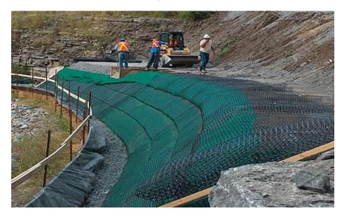
Plate 9.10 - Geogrids being placed on face of slope
