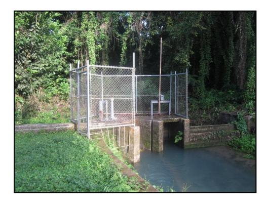
Plate 4.10 - Sluice gate implemented within the channel of Roaring River
