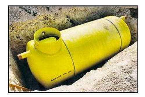
Plate 9.2- Filling station forecourt separator
