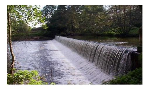
*Plate 9.4 - Example of weir which may be used in conjunction with a detention pond*
