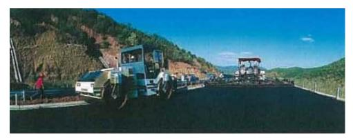
Plate 2.4 - Spreading and Compacting Asphalt Mixture (source CHEC)
