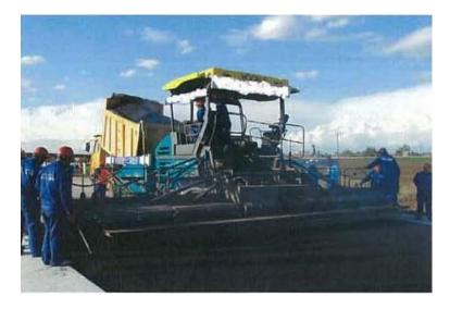
Plate 2.3 - Asphalt Concrete Spreading (source CHEC)
