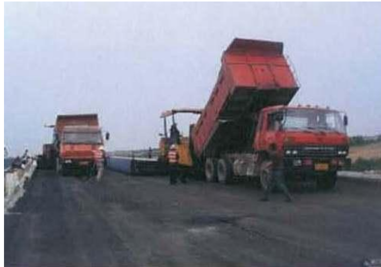
Plate 2.2 - Transportation of Asphalt Concrete (source CHEC)
