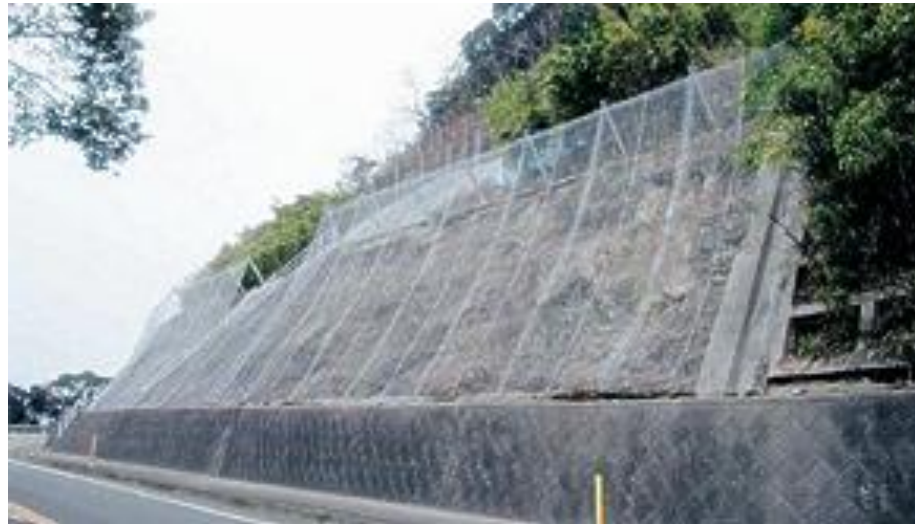
Plate 9.1 - Rockfall catchment fences being implemented
