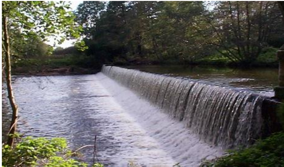
Plate 9.4 - Example of weir which may be used in conjunction with a detention pond
