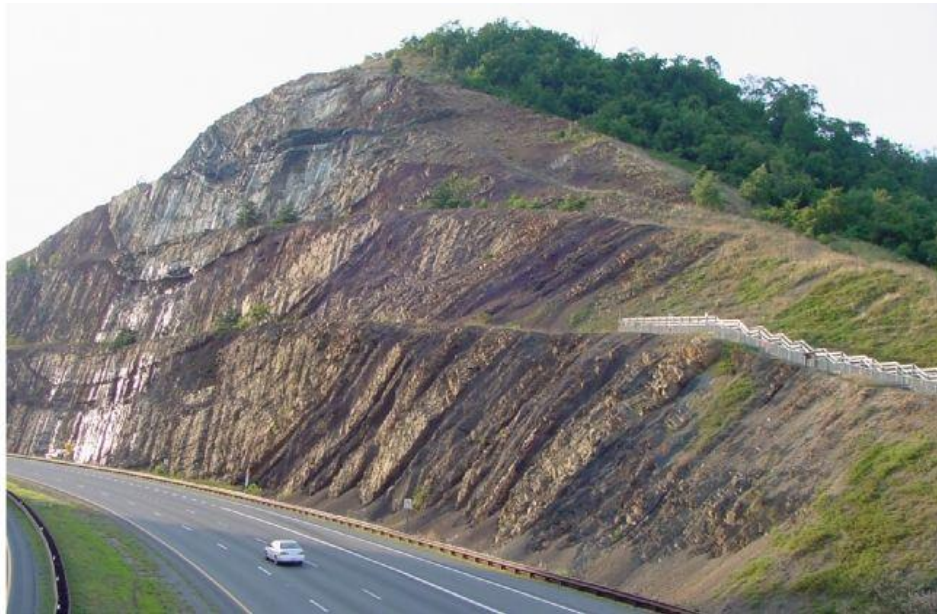
Plate 9.7 - Bench trail cut on face of steep slope
