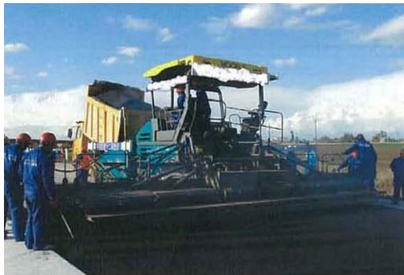
Plate 2.3 -Asphalt Concrete Spreading (source CHEC)
