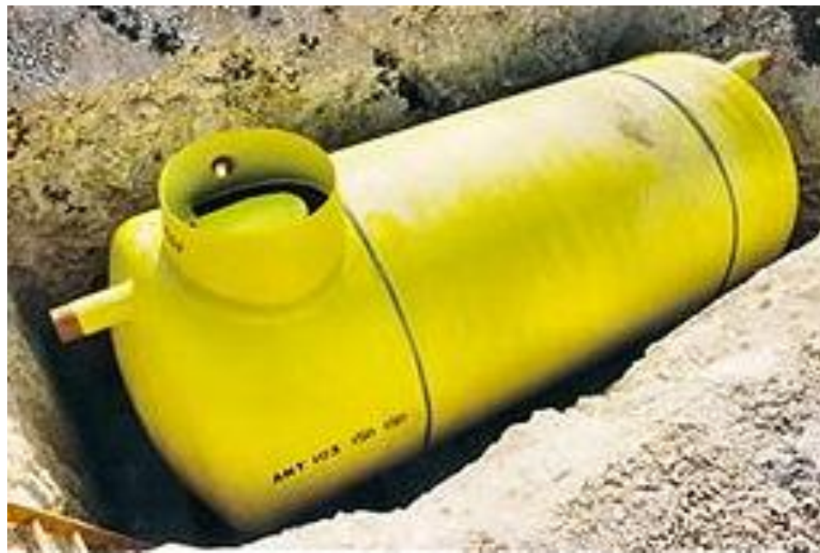
Plate 9.2 - Filling station forecourt separator
