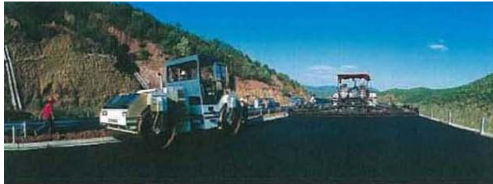
Plate 2.4 - Spreading and Compacting Asphalt Mixture (source CHEC)
