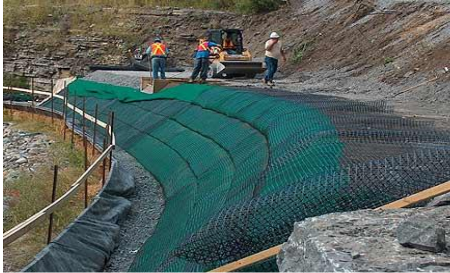
Plate 9.10 - Geogrids being placed on face of slope
