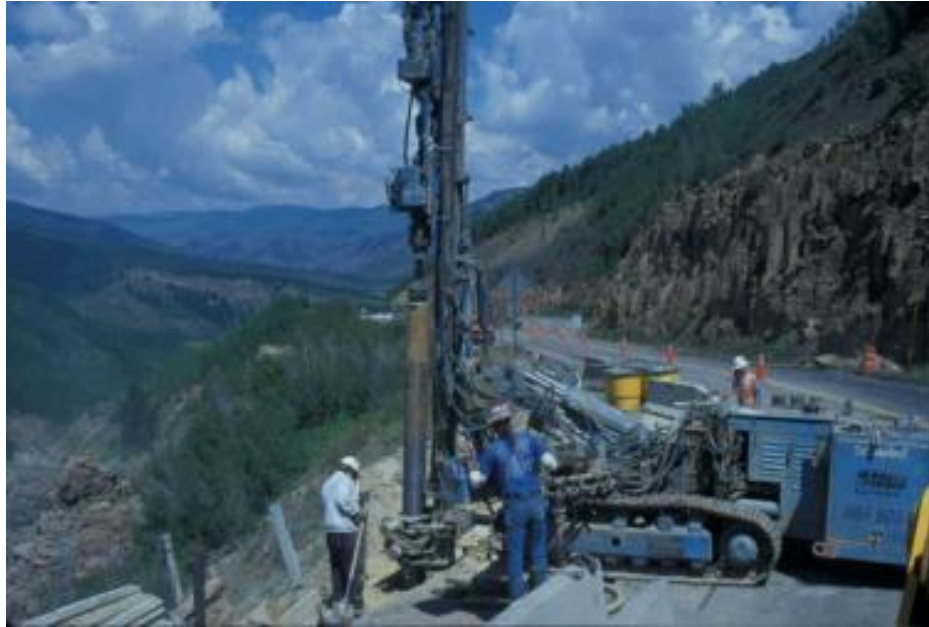
Plate 9.6 - Installation of metal soil nails at edge of slope
