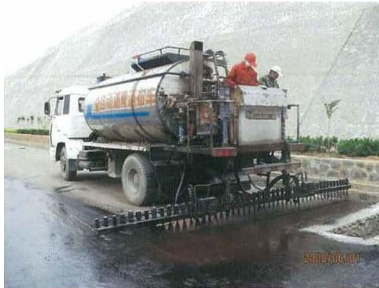
Plate 2.1 - Asphalt Pavement Construction (Spraying) (source CHEC)
