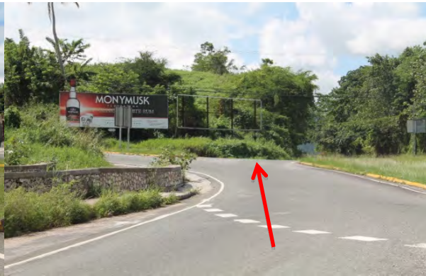
Fig 66. This roundabout poses no issues for maneuvering, as the corners are long and not sharp. The curbs are also low and the rear wheels can cross over the islands.
