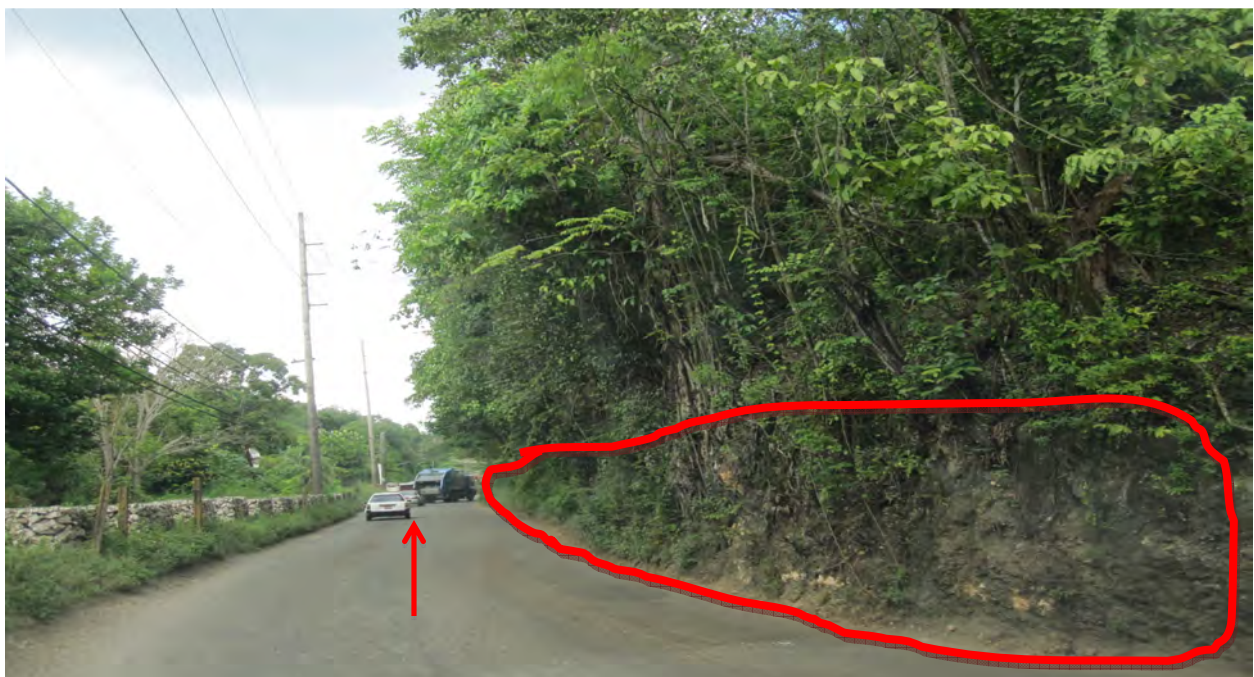
Fig 57. 20 feet of limestone and existing trees as shown in the picture must be excavated in order to create a passage for the trailers. This will entail negotiating with the national works agency to have this conducted and also put plans in place for traffic control when this is to be done.
