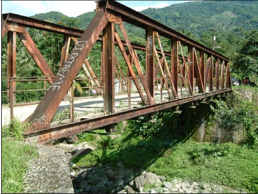
Figure 1: 4 Typical Timber Deck Bailey bridge
