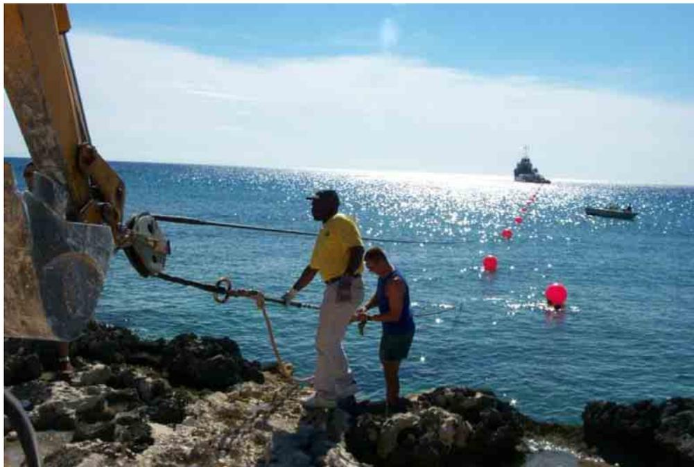
**FIGURE 1-18: ILLUSTRATION OF INSTALLATION FROM SHIP WITH A SHEAVE**
