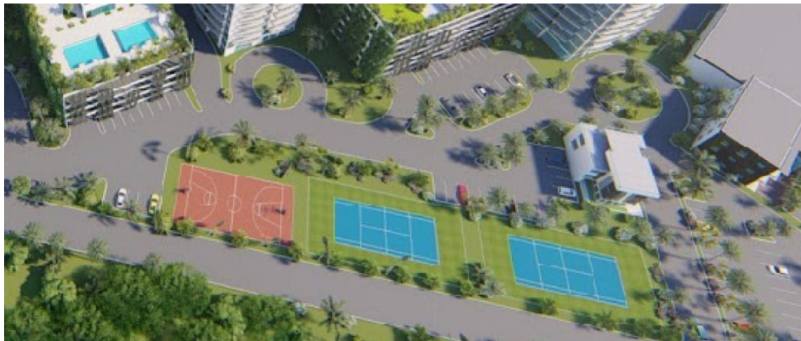
Plate 3-7 View of Amenities Area
