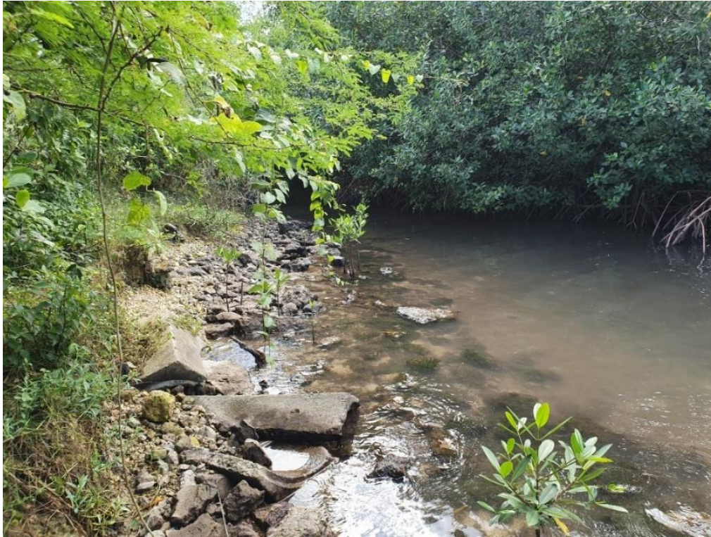
Plate 4-16 Narrow creek (northern end) separating proposed development site from Western mangroves- with historically placed rubble and fill material evident
