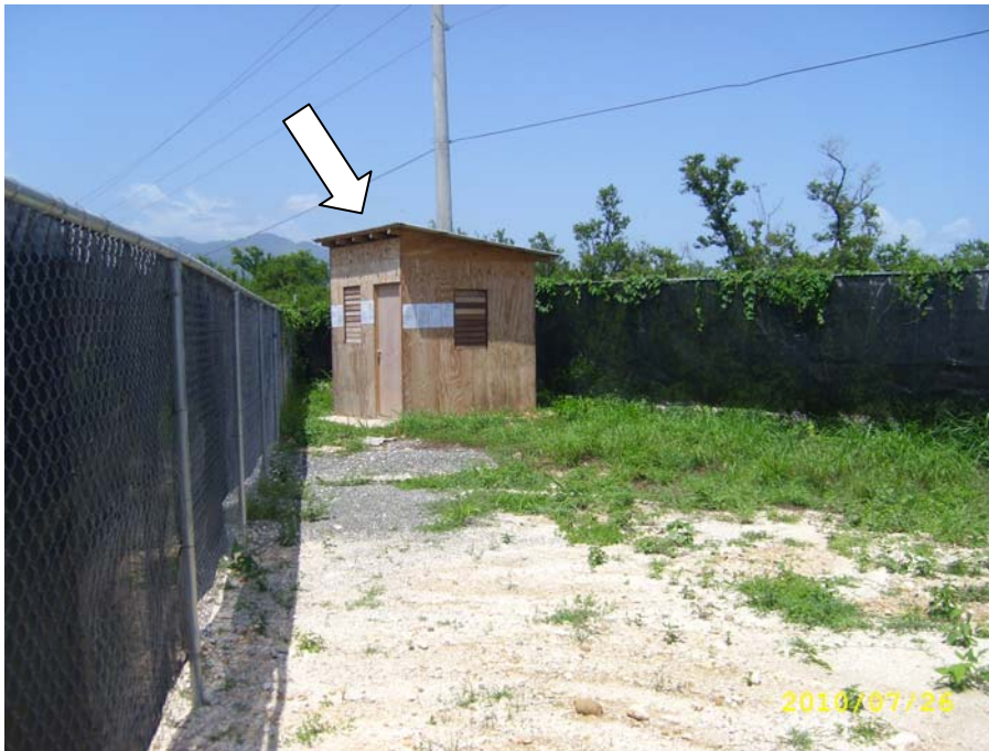
Plate 5 Photo showing storage shed
