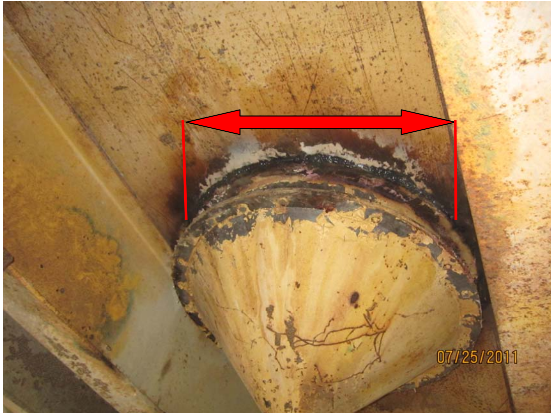
Plate 3 Photo showing where welding occurred
