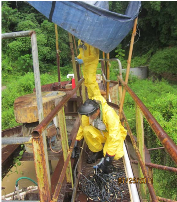
Plate 18 Photo showing sampling of Tank T1
