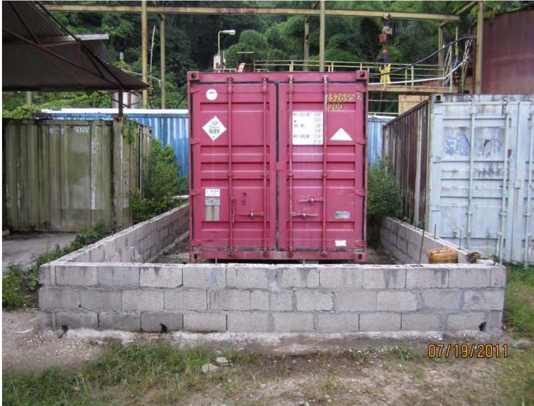
Plate 12 Photo showing container with sodium cyanide pellets surrounded by concrete wall
