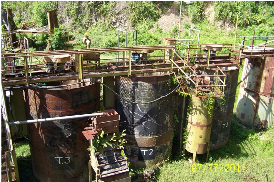
Plate 2 Photo showing smaller tanks T0, T1, T2, T3 and T4 (out of view)
