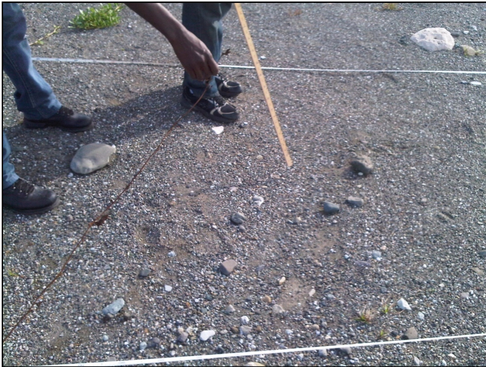
Plate 4 Drainage grooves in area of plant mortality in Transect 1
